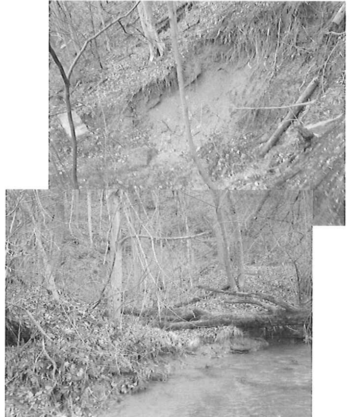
Current Shinns Run site for the WV DEP project.
