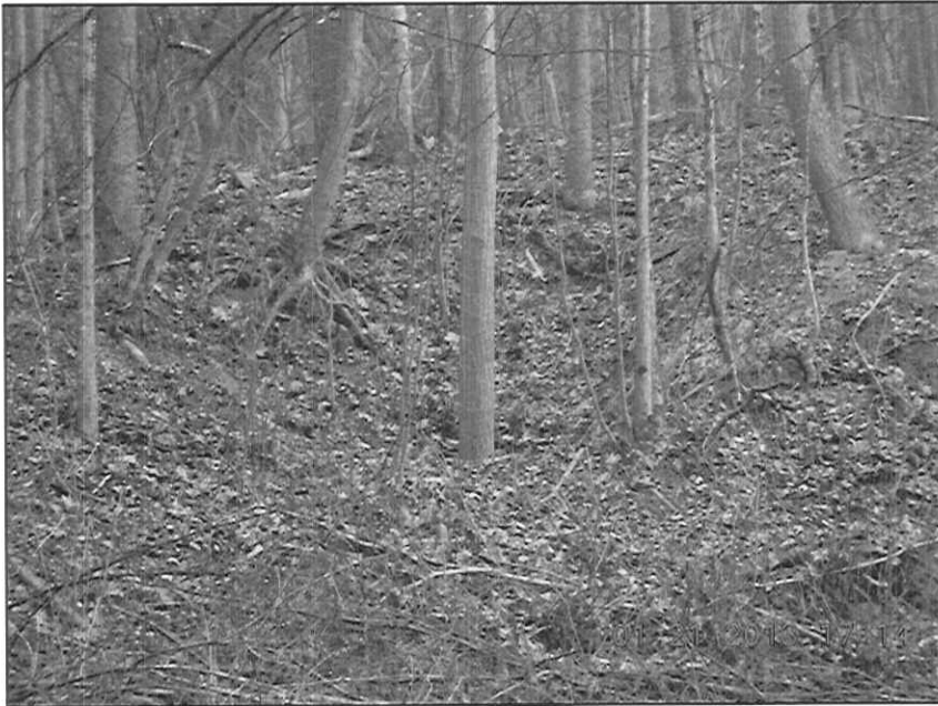
Photo D – Shinns Run – Subsidence Feature
