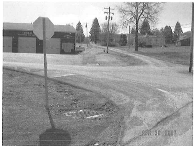
New Storm Drains and Catch Basins
