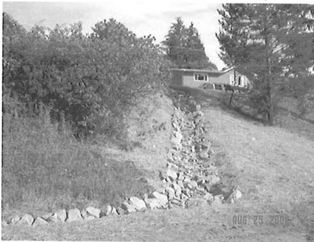
Erosion Repair – Rip Rap Armored Ditch
