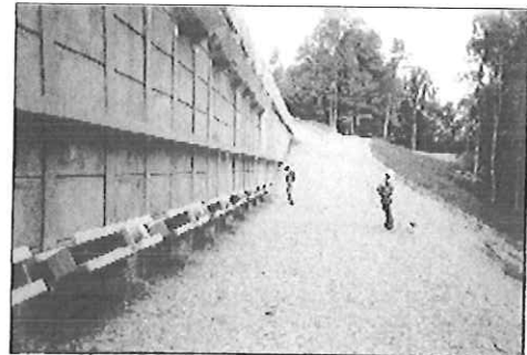
Finished wall with anchors
