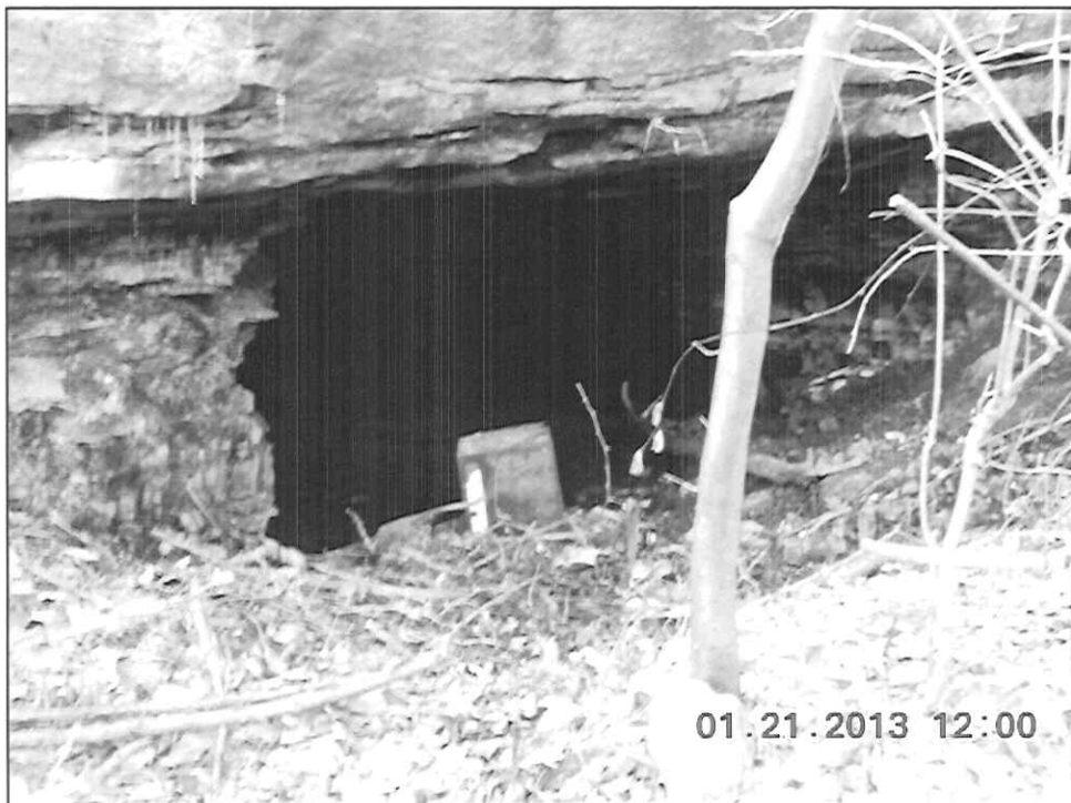
Photo C – Site 2, Open Portal at Highwall
