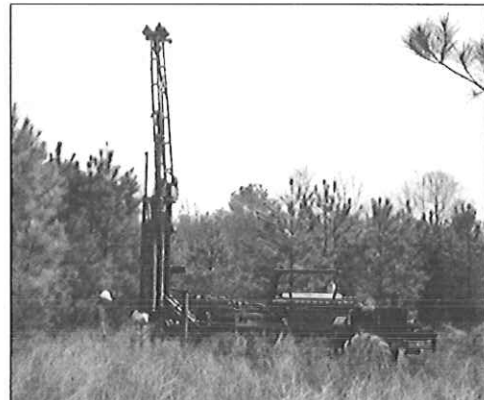
CTL's ATV can drill in rough terrain
