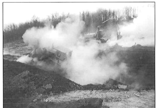
Jamison Burning Refuse Reclamation Project
