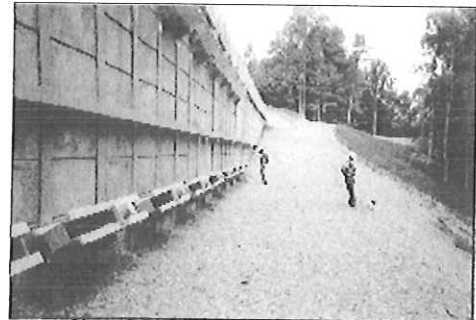
Finished wall with anchors
