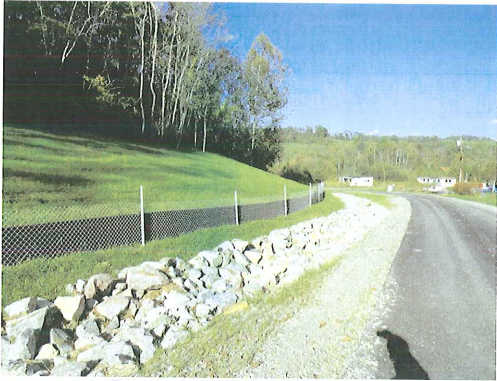
Prospect Valley Highwall #4 – DEP14433
