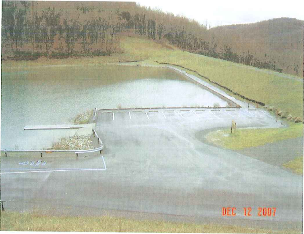
BAILEY DAM MODIFICATION, MONONGALIA CO., WV
