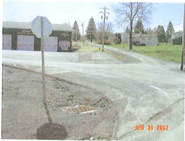
New Storm Drains and Catch Basins
