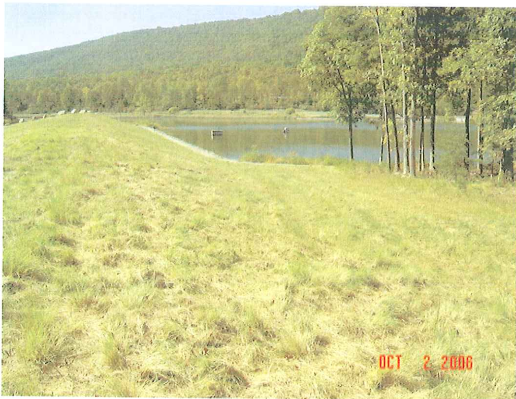
WARDEN LAKE DAM MODIFICATION, HARDY CO., WV
