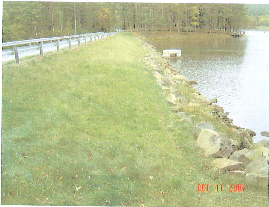
MONCOVE DAM MODIFICATION, MONROE CO., WV
