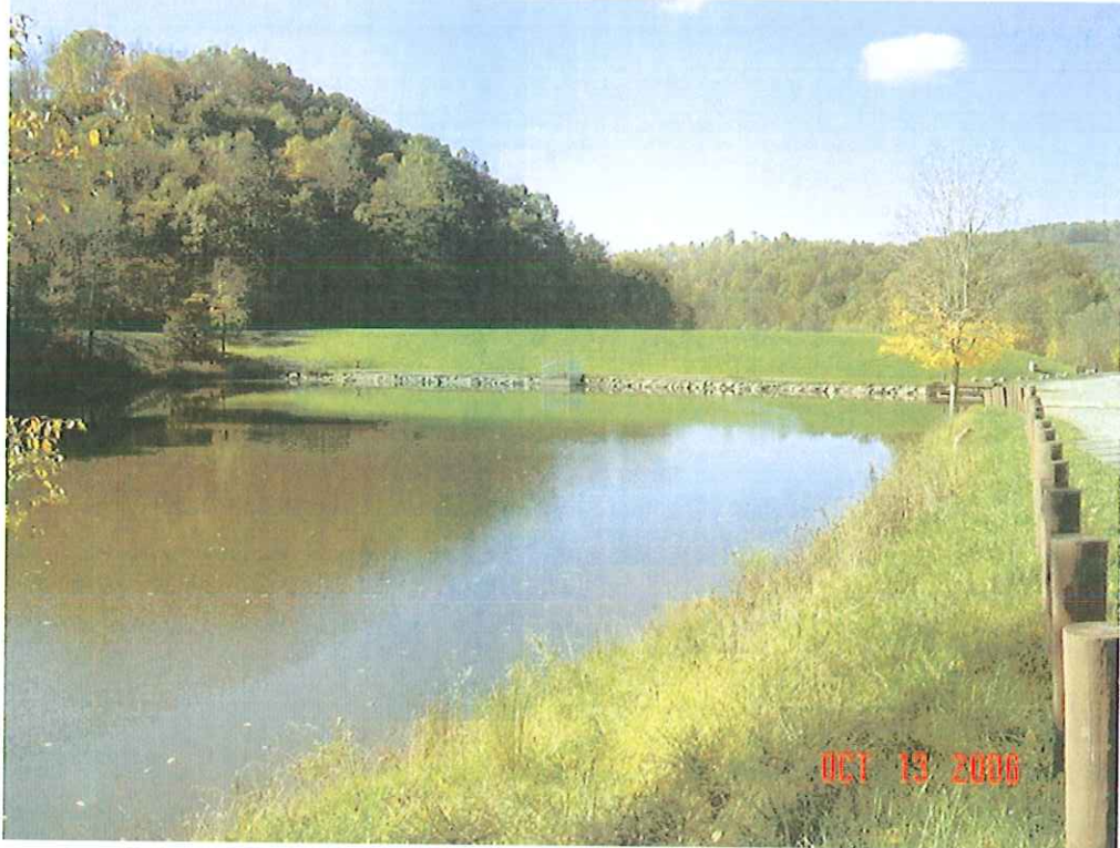
JIMMY LEWIS DAM MODIFICATION, MERCER CO., WV
