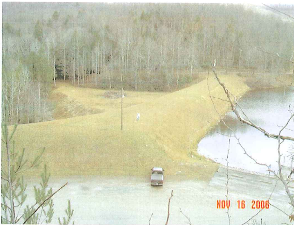
PLUM ORCHARD DAM MODIFICATION, FAYETTE CO., WV
