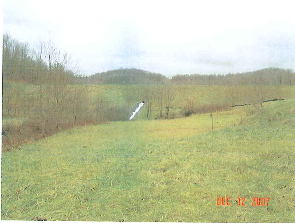
LEMLEY DAM MODIFICATION, MONONGALIA CO., WV
