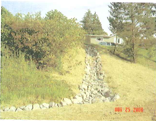
Erosion Repair – Rip Rap Armored Ditch
