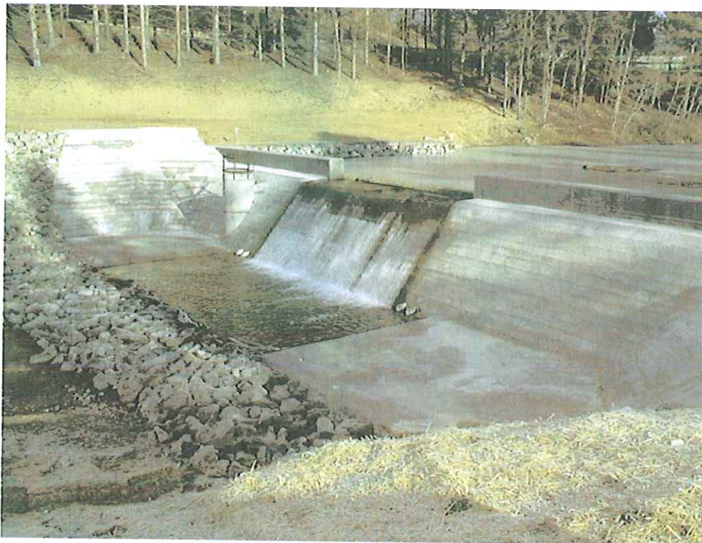
THOMAS DAM MODIFICATION, THOMAS, WV
