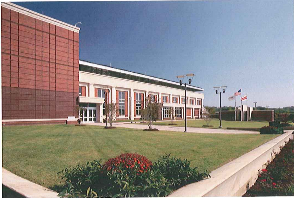
At the Unified Communications Center in Washington DC , site security was addressed with a perimeter fence, but also with a landscape wall that blends into the landscape.
