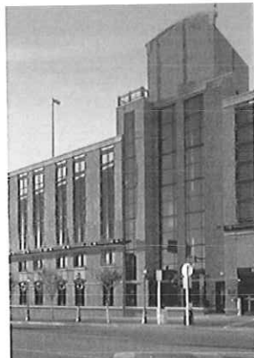
Western Pennsylvania Hospital Parking Garage
