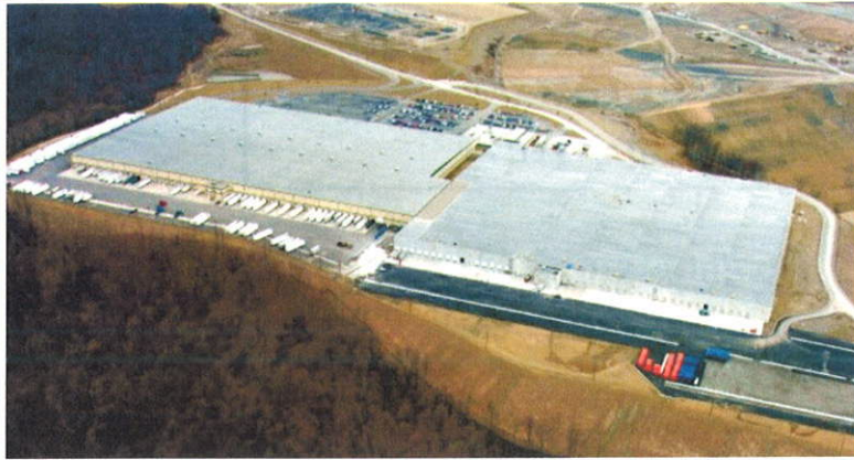
Cabela's Eastern Distribution Center
