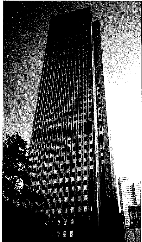
Three Mellon Center. This high-rise was retrofit in the mid-1980's and is currently undergoing a phased modernization program to provide an increased level of reliability for computer operations.
