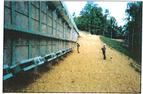
Finished wall with anchors
