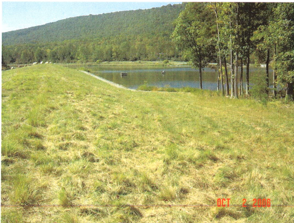
WARDEN LAKE DAM MODIFICATION, HARDY CO., WV
