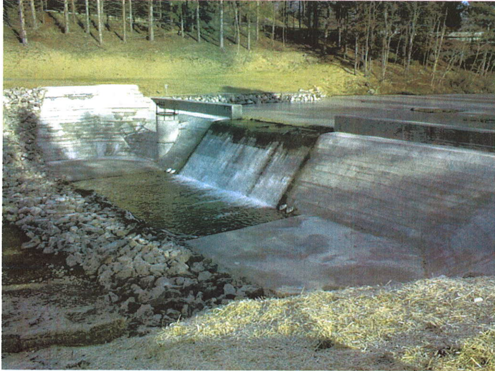
THOMAS DAM MODIFICATION, THOMAS, WV
