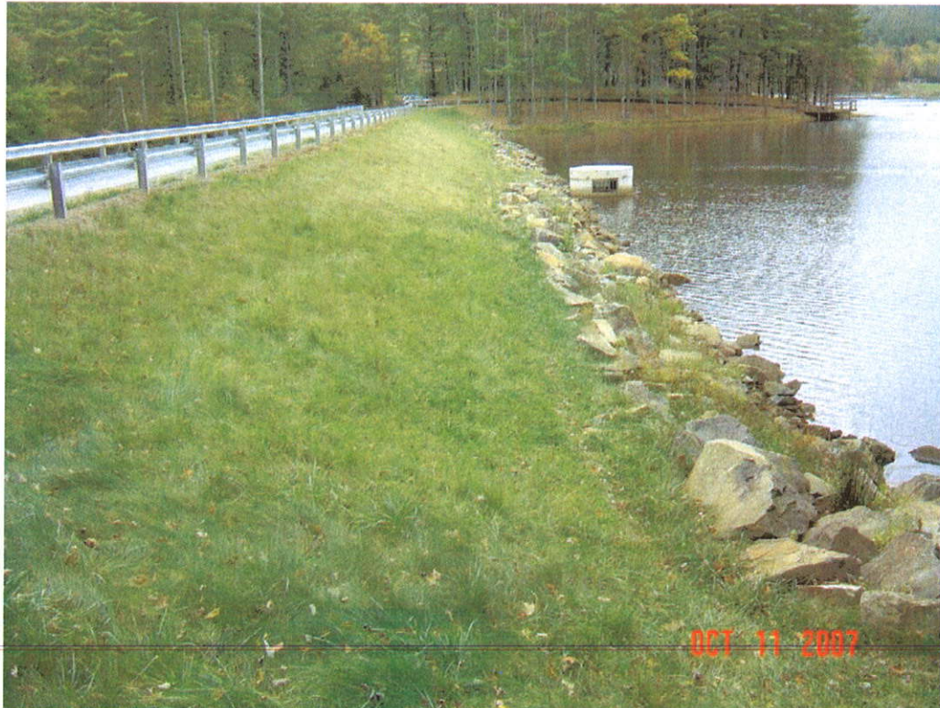
MONCOVE DAM MODIFICATION, MONROE CO., WV
