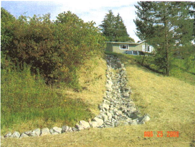
Erosion Repair – Rip Rap Armored Ditch
