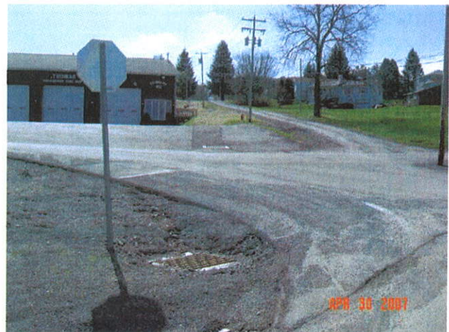
New Storm Drains and Catch Basins
