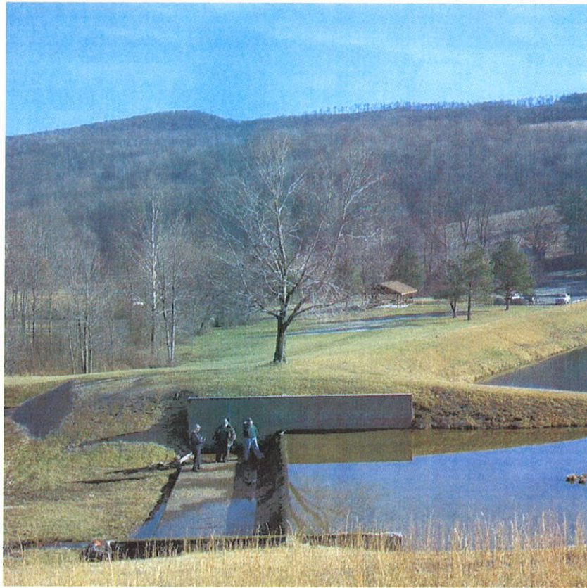
BELINGTON DAM MODIFICATION, BELINGTON, WV
