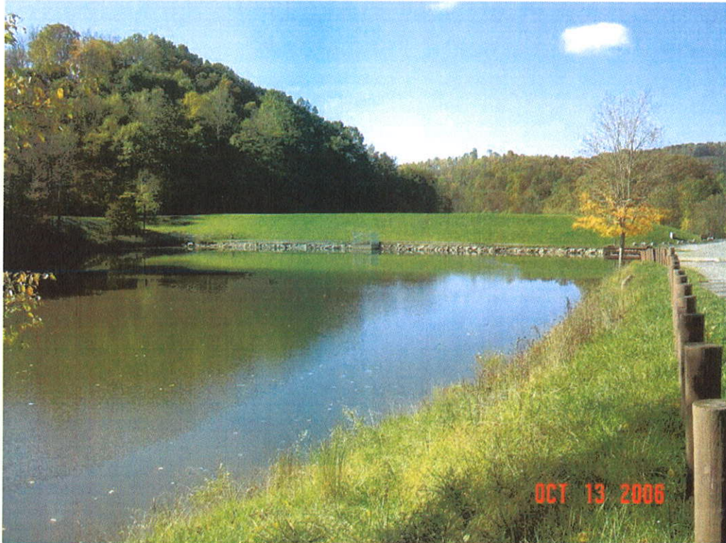
JIMMY LEWIS DAM MODIFICATION, MERCER CO., WV
