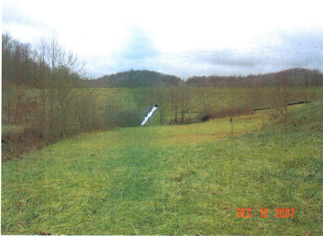
LEMLEY DAM MODIFICATION, MONONGALIA CO., WV
