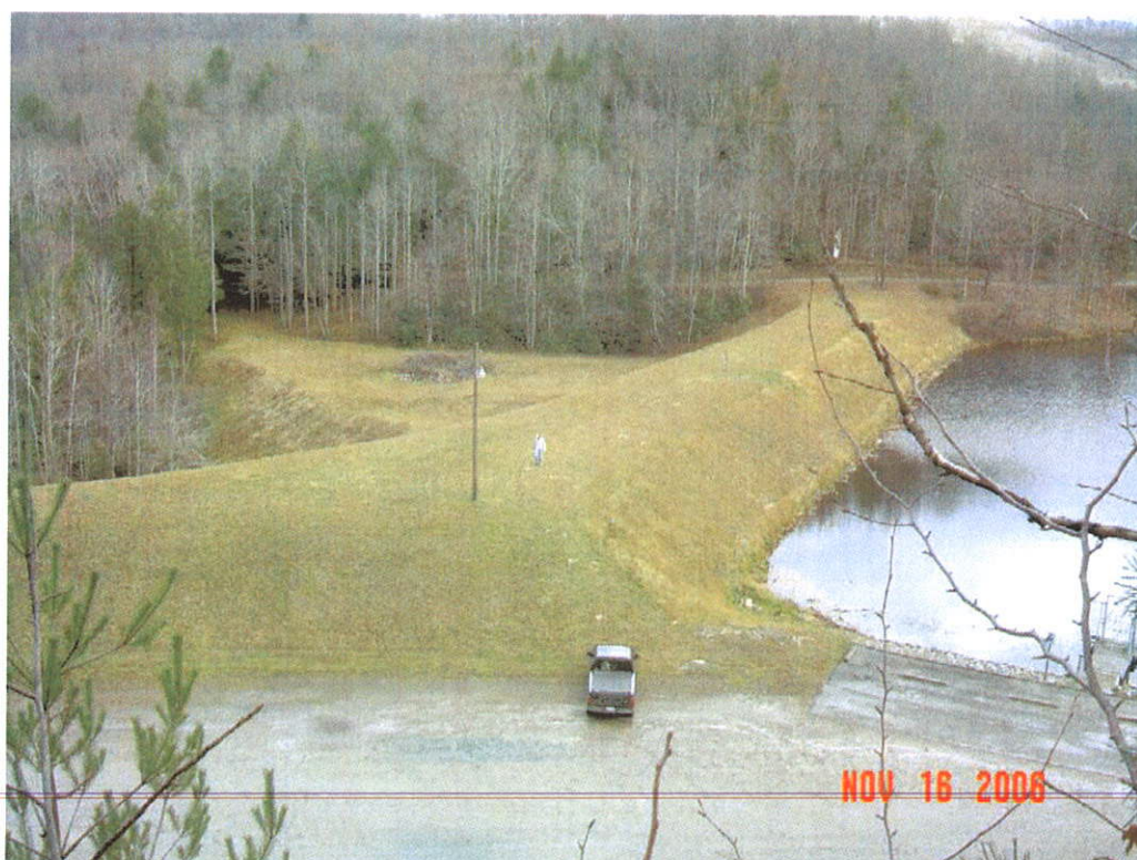
PLUM ORCHARD DAM MODIFICATION, FAYETTE CO., WV
