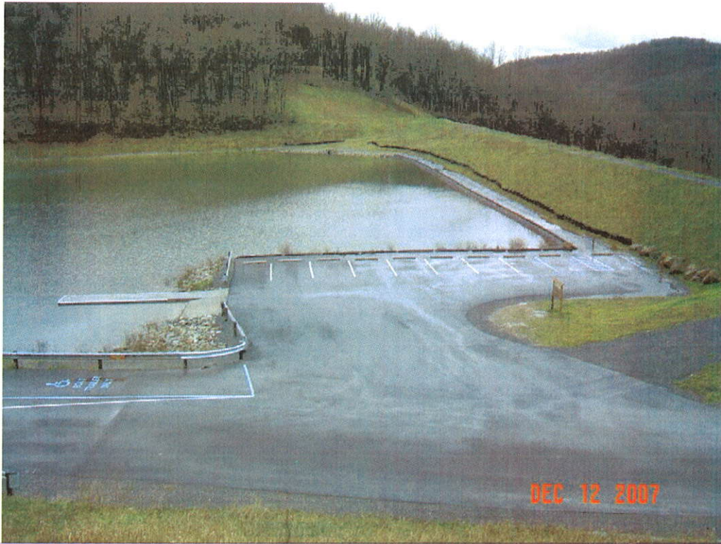
BAILEY DAM MODIFICATION, MONONGALIA CO., WV
