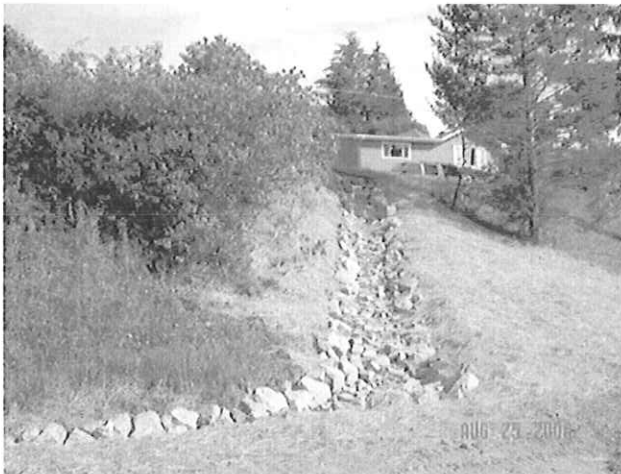
Erosion Repair – Rip Rap Armored Ditch
