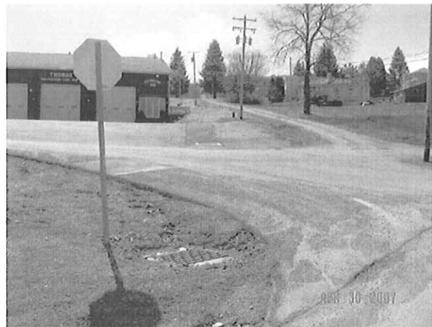
New Storm Drains and Catch Basins
