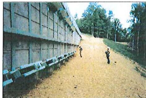
Finished wall with anchors
