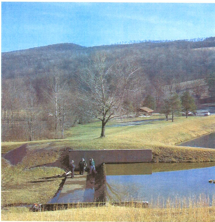
BELINGTON DAM MODIFICATION, BELINGTON, WV
