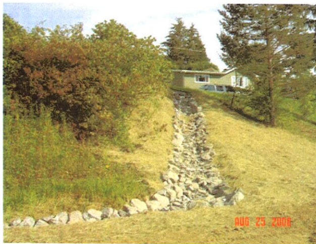
Erosion Repair – Rip Rap Armored Ditch
