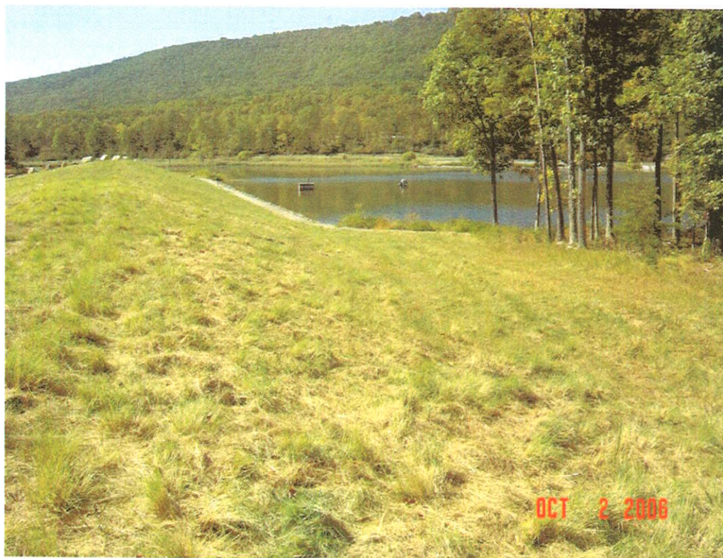
WARDEN LAKE DAM MODIFICATION, HARDY CO., WV
