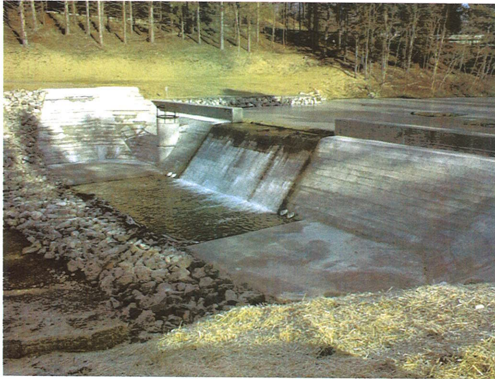
THOMAS DAM MODIFICATION, THOMAS, WV
