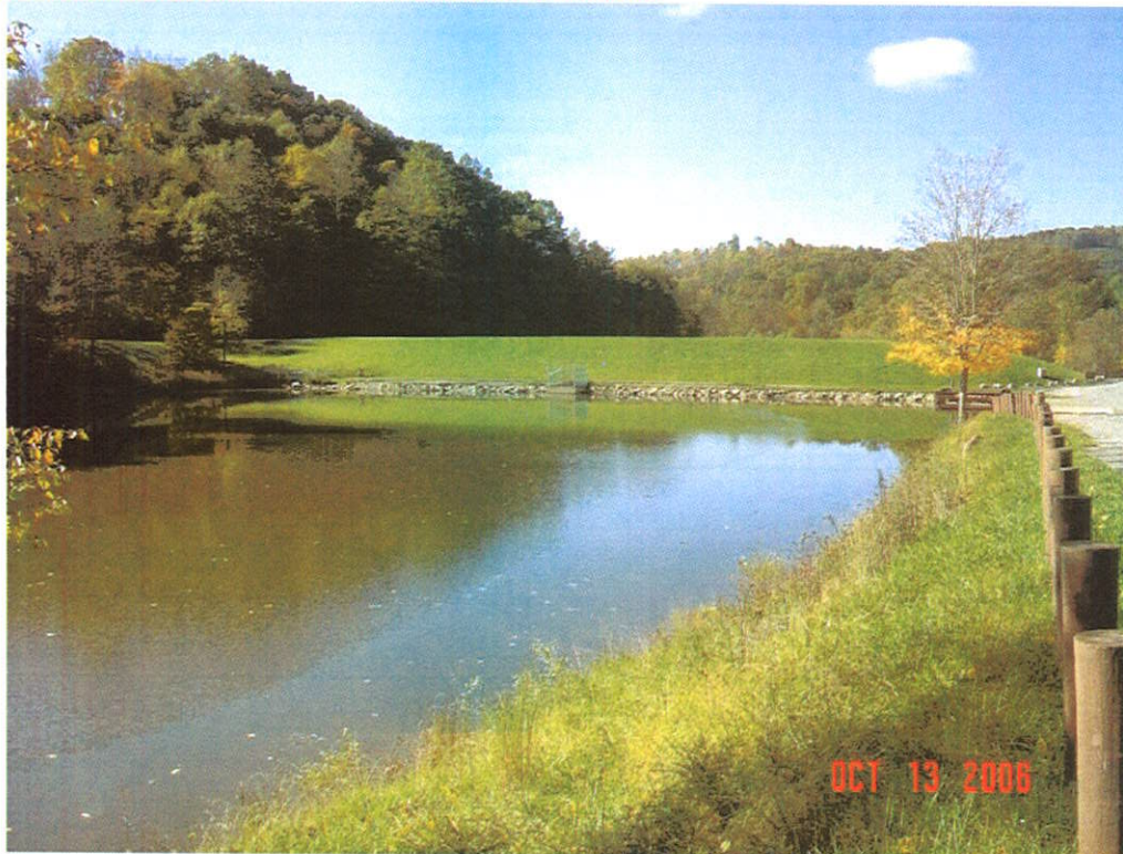
JIMMY LEWIS DAM MODIFICATION, MERCER CO., WV
