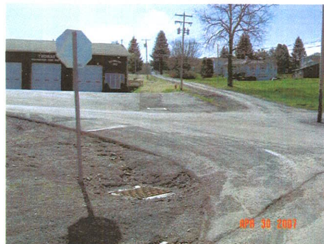
New Storm Drains and Catch Basins
