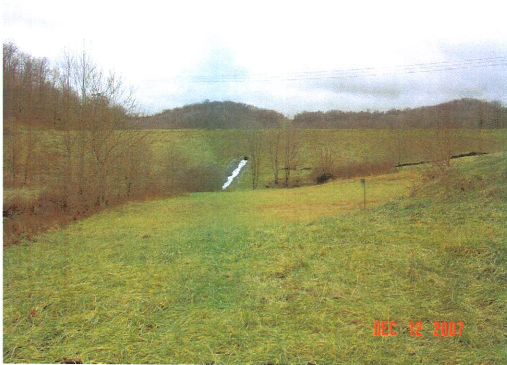
LEMLEY DAM MODIFICATION, MONONGALIA CO., WV
