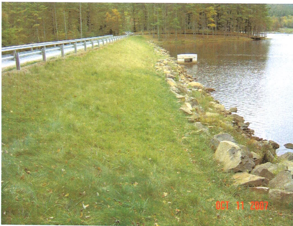
MONCOVE DAM MODIFICATION, MONROE CO., WV
