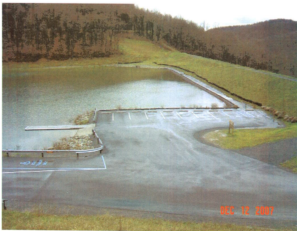
BAILEY DAM MODIFICATION, MONONGALIA CO., WV
