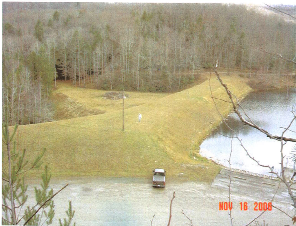
PLUM ORCHARD DAM MODIFICATION, FAYETTE CO., WV
