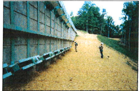
Finished wall with anchors
