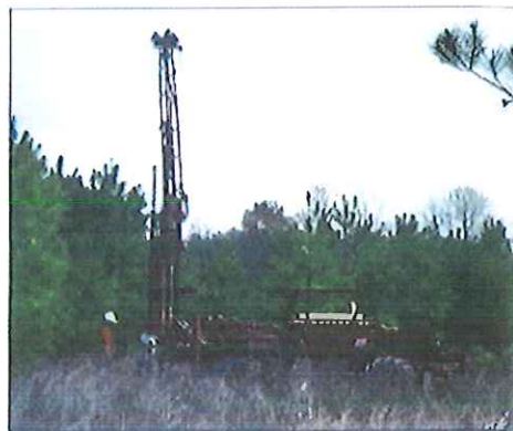
CTL's ATV can drill in rough terrain
