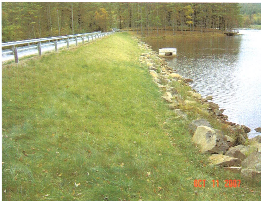
MONCOVE DAM MODIFICATION, MONROE CO., WV
