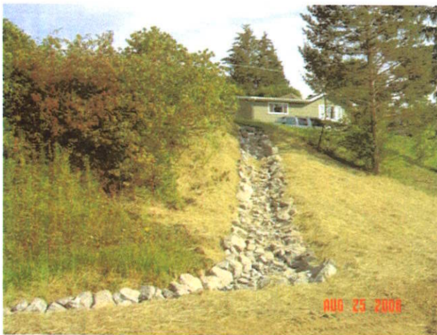
Erosion Repair – Rip Rap Armored Ditch
