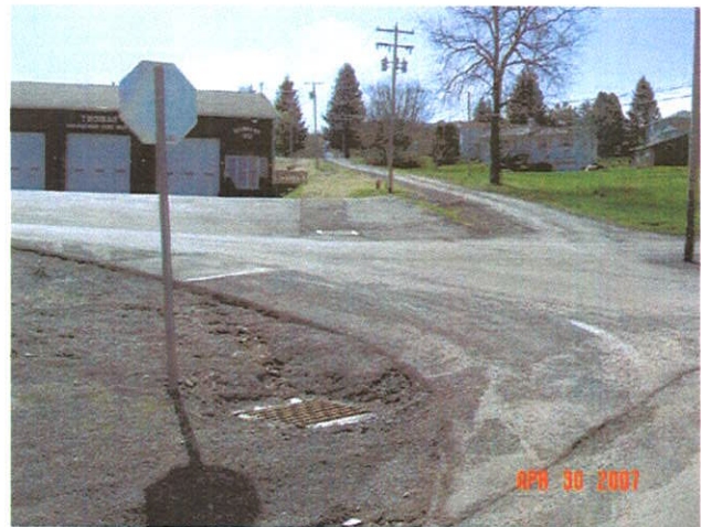
New Storm Drains and Catch Basins
