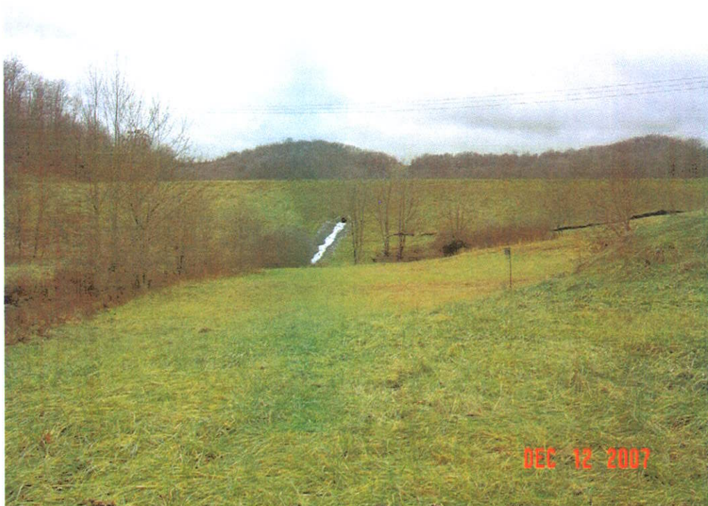
LEMLEY DAM MODIFICATION, MONONGALIA CO., WV
