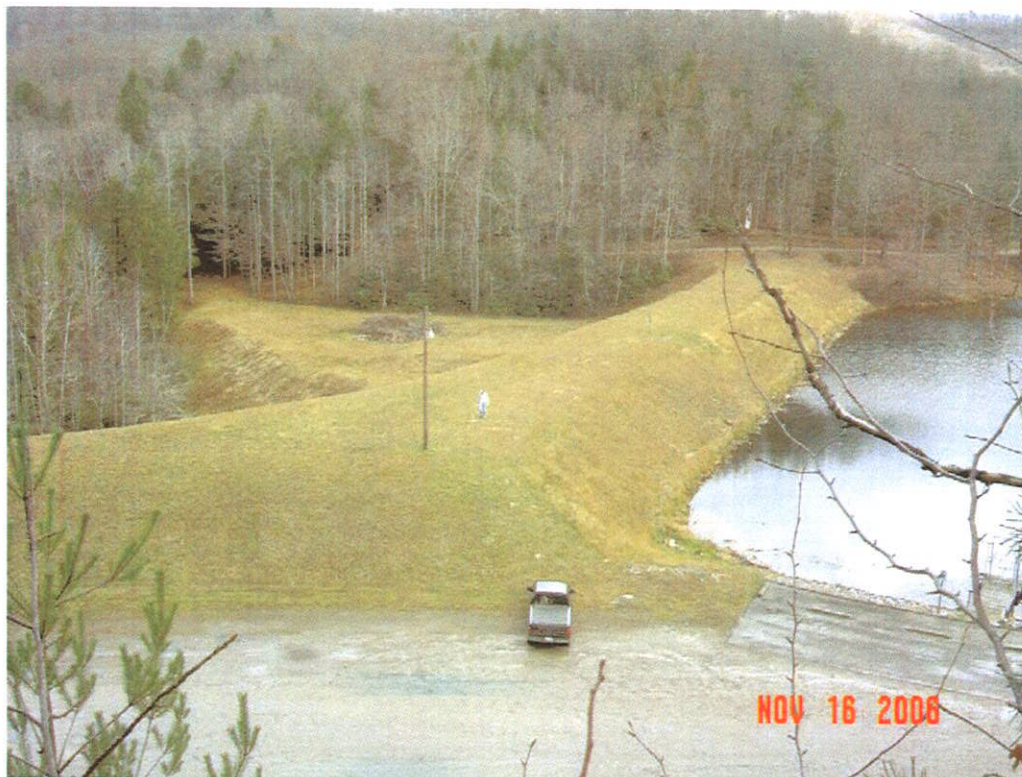
PLUM ORCHARD DAM MODIFICATION, FAYETTE CO., WV
