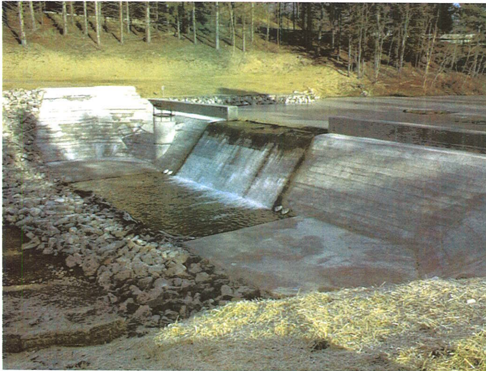
THOMAS DAM MODIFICATION, THOMAS, WV
