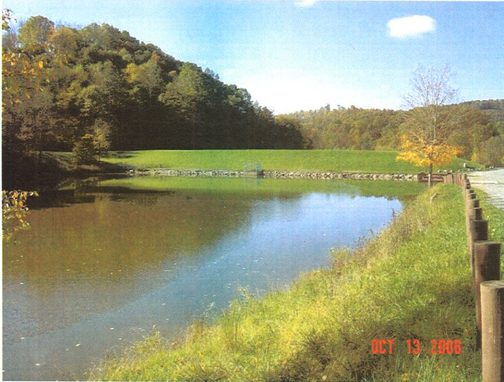
JIMMY LEWIS DAM MODIFICATION, MERCER CO., WV
