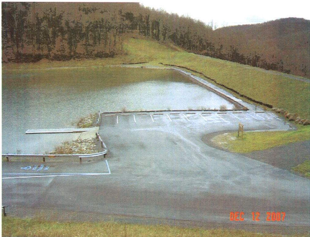
BAILEY DAM MODIFICATION, MONONGALIA CO., WV
