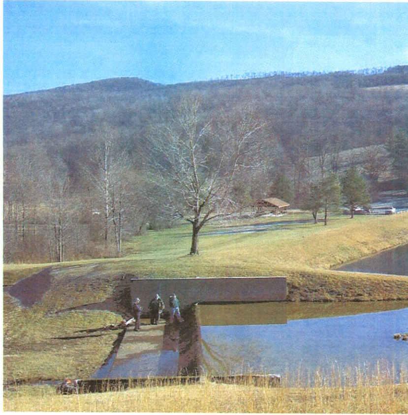
BELINGTON DAM MODIFICATION, BELINGTON, WV
