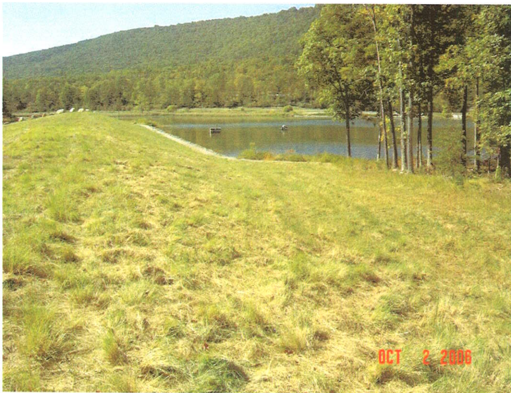
WARDEN LAKE DAM MODIFICATION, HARDY CO., WV
