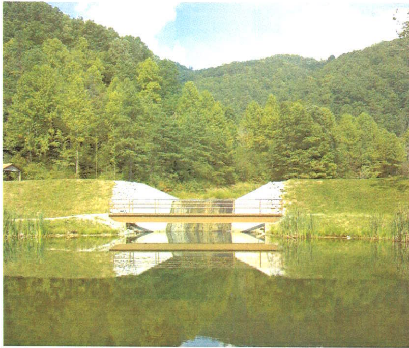
OLD ANAWALT DAM FLOOD DAMAGE REPAIR, MCDOWELL CO., WV
