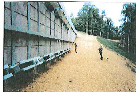
Finished wall with anchors
