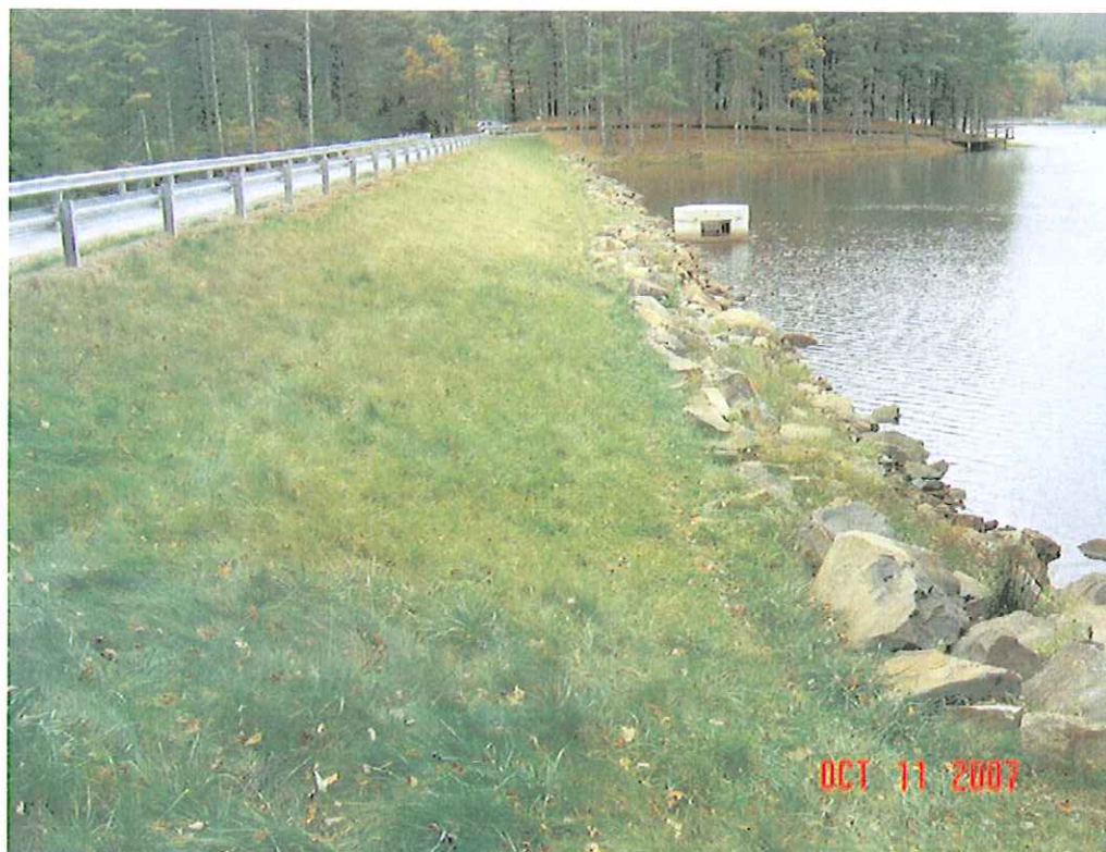
MONCOVE DAM MODIFICATION, MONROE CO., WV
