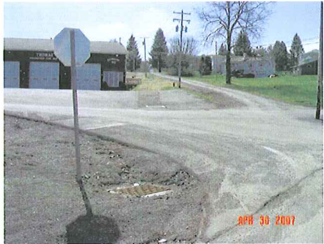
New Storm Drains and Catch Basins
