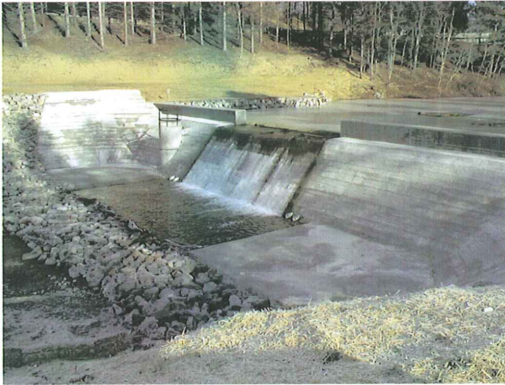
THOMAS DAM MODIFICATION, THOMAS, WV
