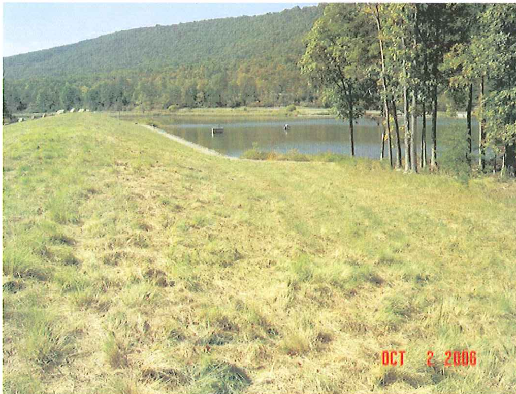
WARDEN LAKE DAM MODIFICATION, HARDY CO., WV
