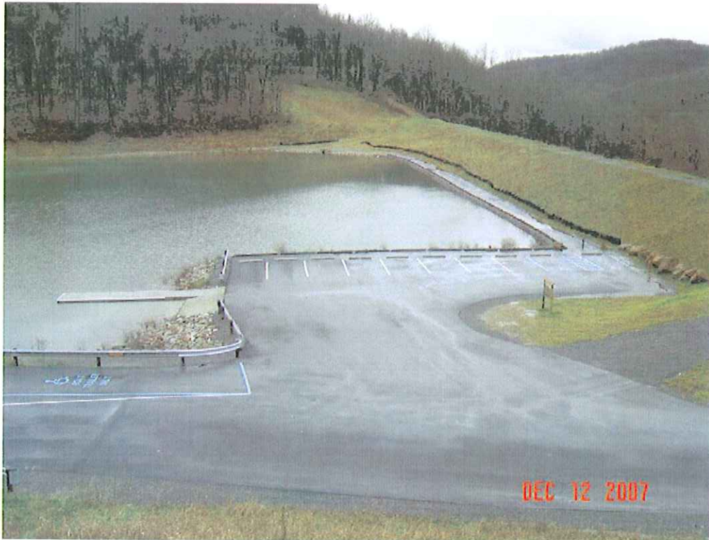
BAILEY DAM MODIFICATION, MONONGALIA CO., WV
