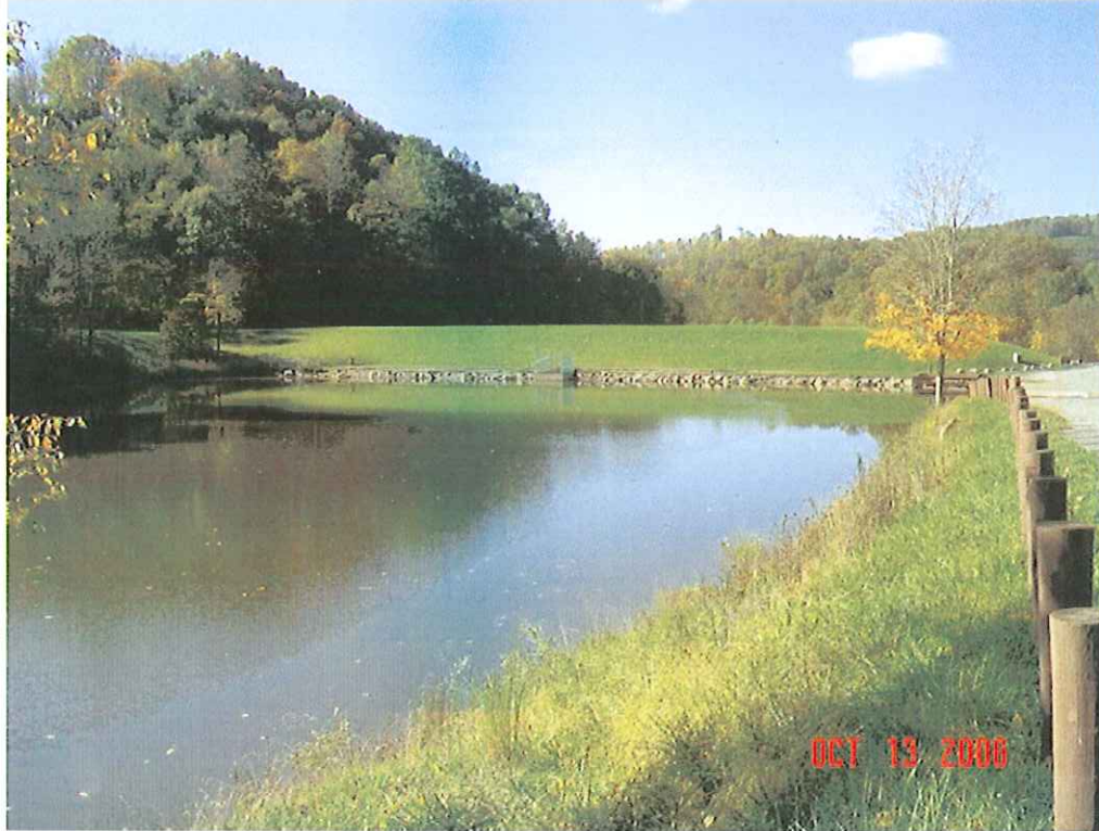
JIMMY LEWIS DAM MODIFICATION, MERCER CO., WV
