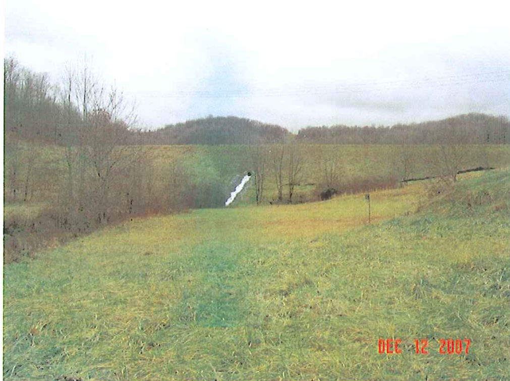
LEMLEY DAM MODIFICATION, MONONGALIA CO., WV
