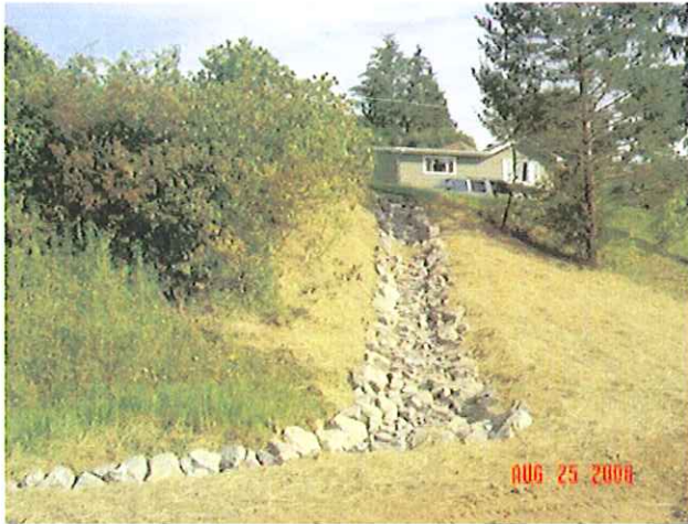
Erosion Repair – Rip Rap Armored Ditch
