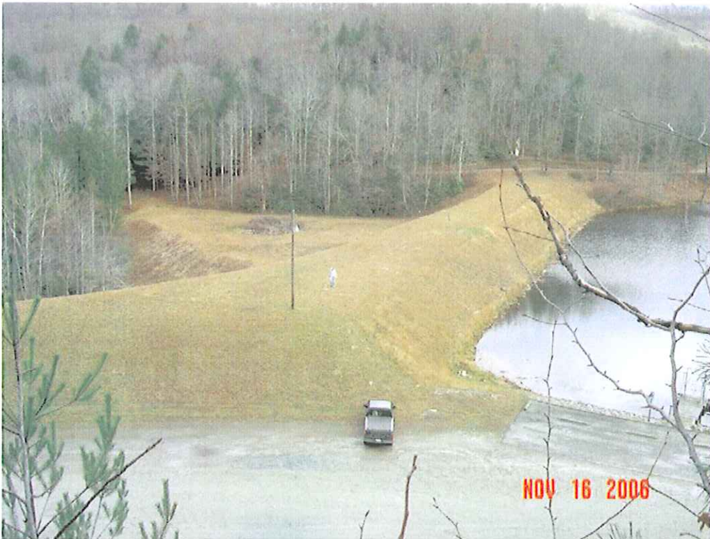
PLUM ORCHARD DAM MODIFICATION, FAYETTE CO., WV
