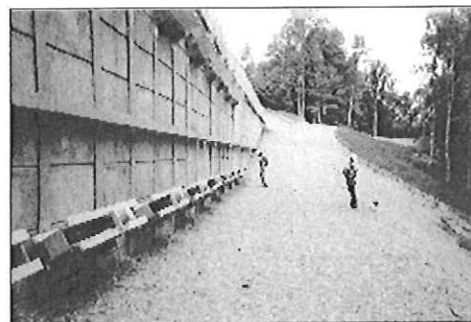
Finished wall with anchors
