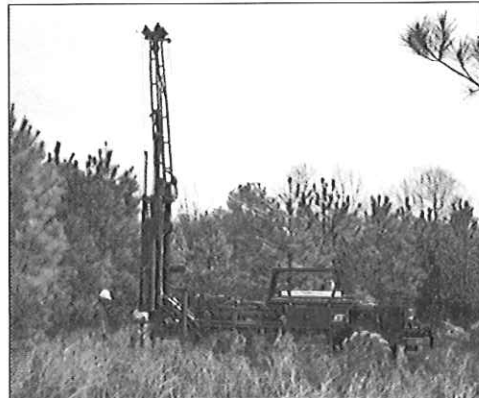
CTL's ATV can drill in rough terrain
