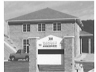
Thrasher Engineering, Inc. Office – Charleston, WV
