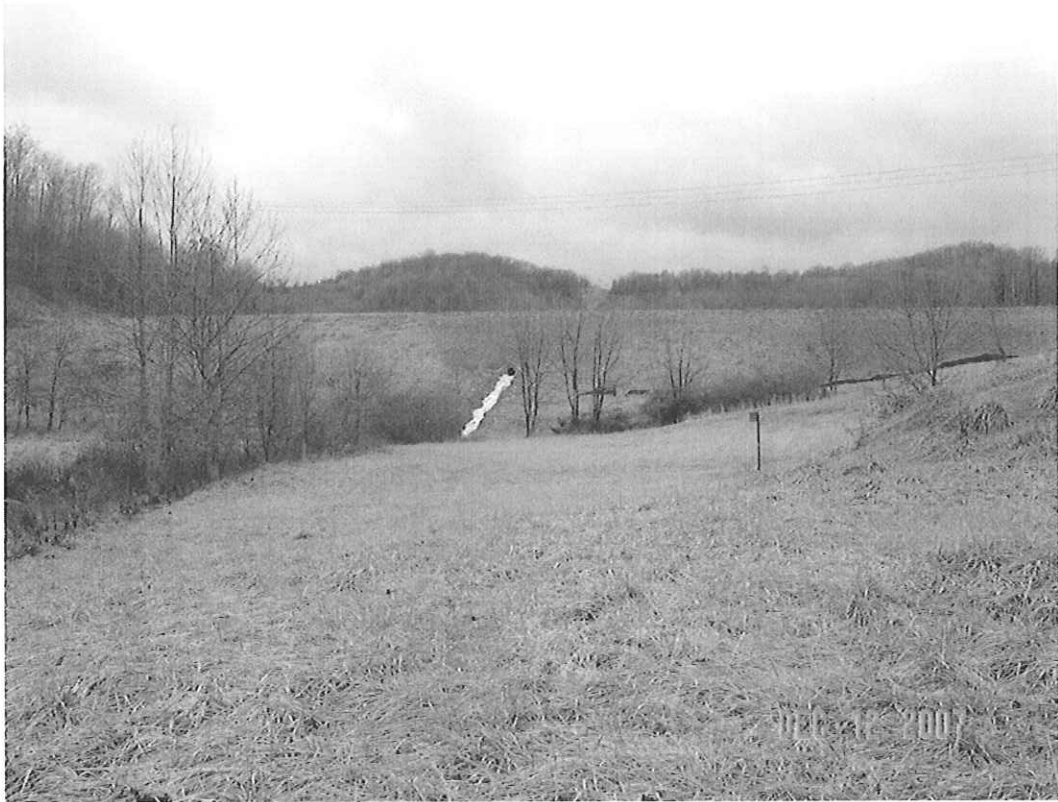
LEMLEY DAM MODIFICATION, MONONGALIA CO., WV
