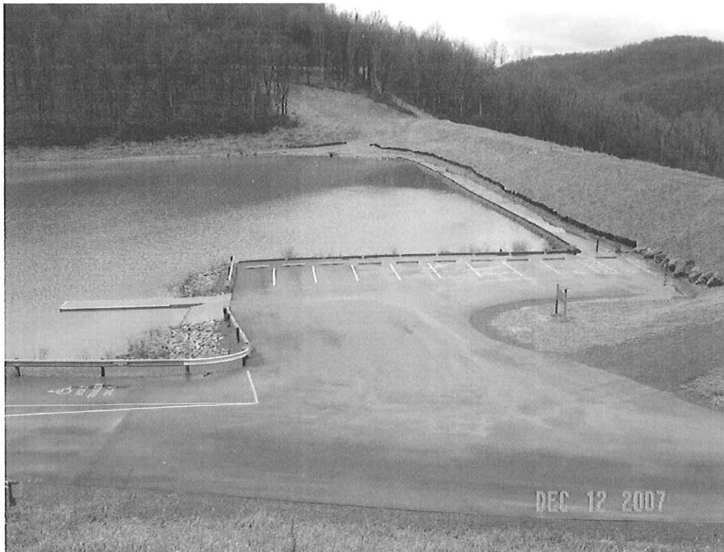
BAILEY DAM MODIFICATION, MONONGALIA CO., WV
