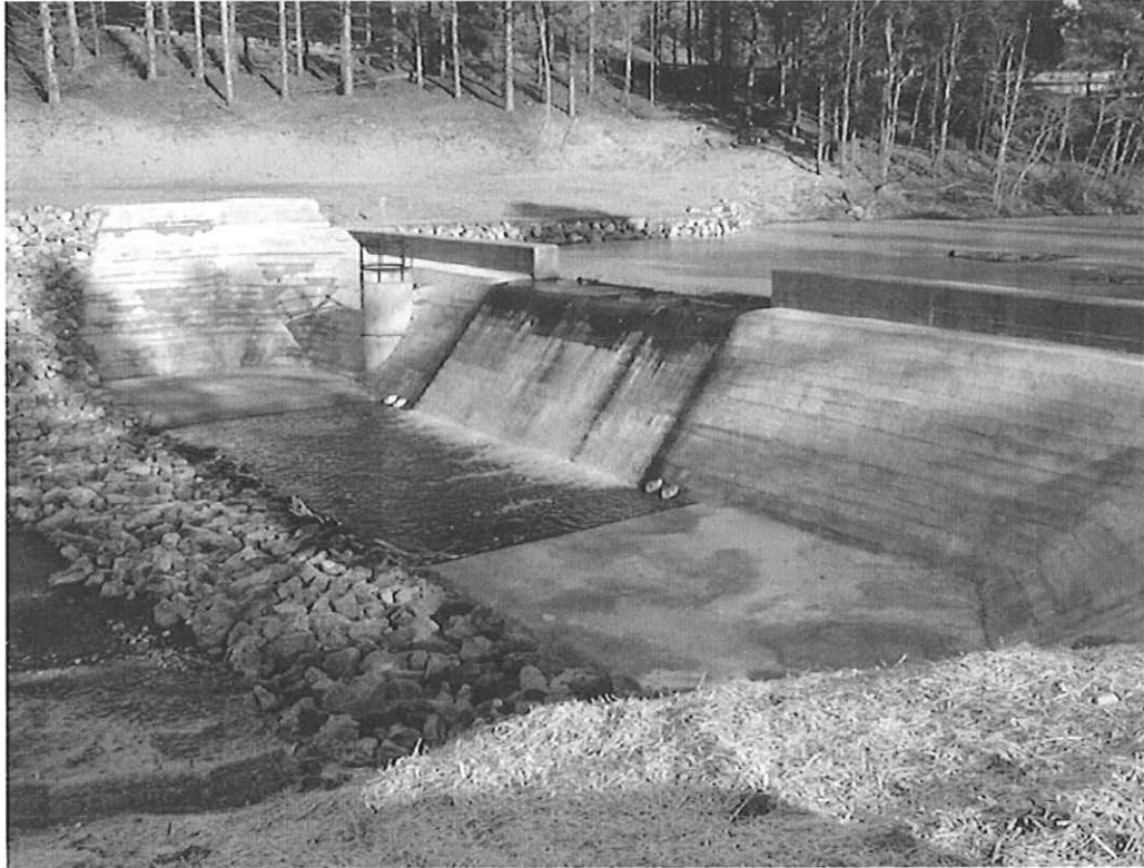
THOMAS DAM MODIFICATION, THOMAS, WV
