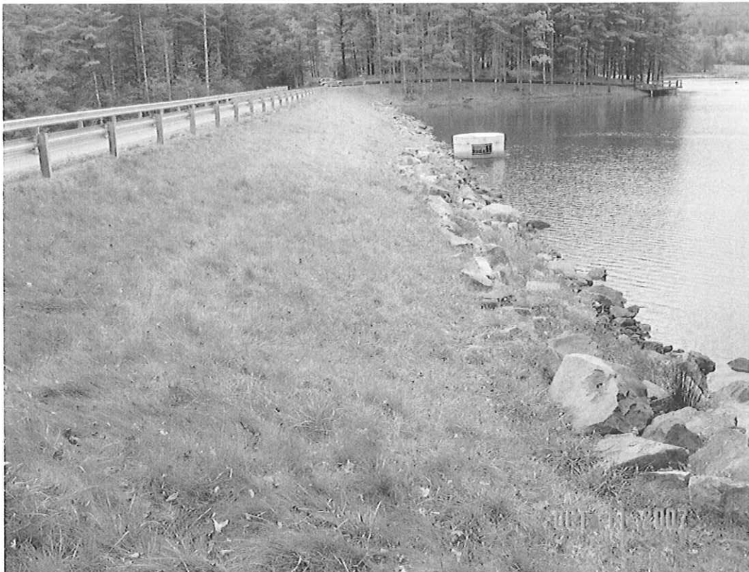
MONCOVE DAM MODIFICATION, MONROE CO., WV
