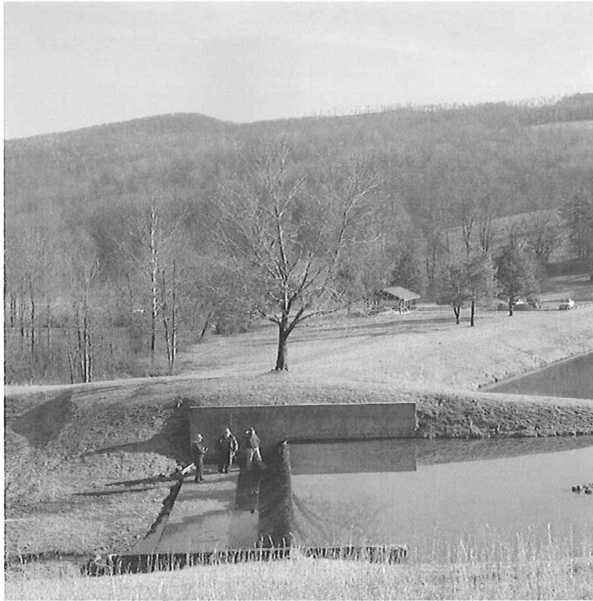
BELINGTON DAM MODIFICATION, BELINGTON, WV
