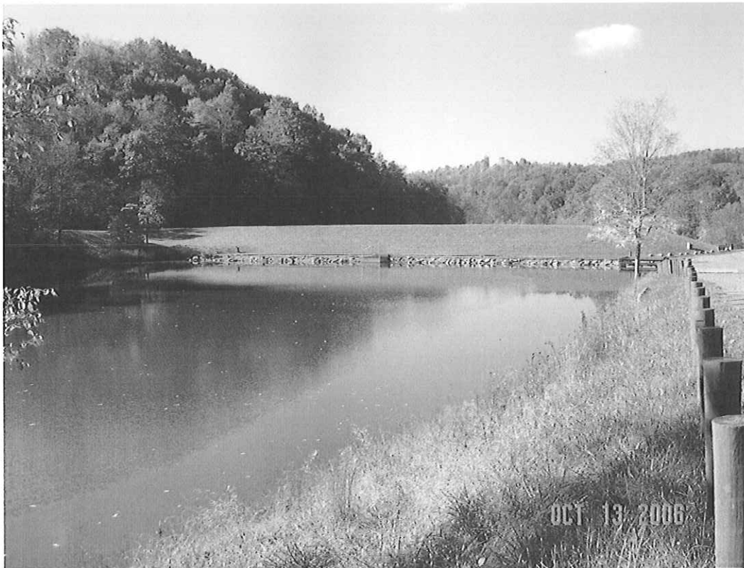
JIMMY LEWIS DAM MODIFICATION, MERCER CO., WV
