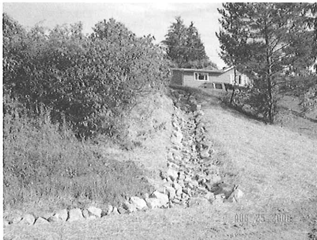
Erosion Repair – Rip Rap Armored Ditch
