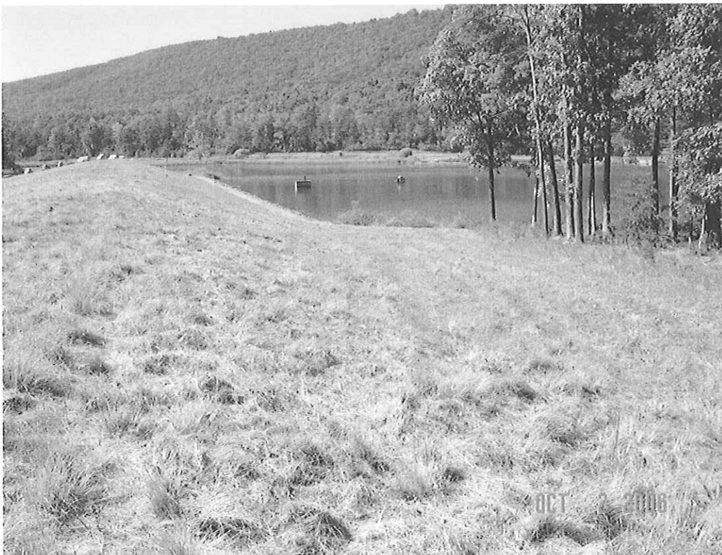
WARDEN LAKE DAM MODIFICATION, HARDY CO., WV
