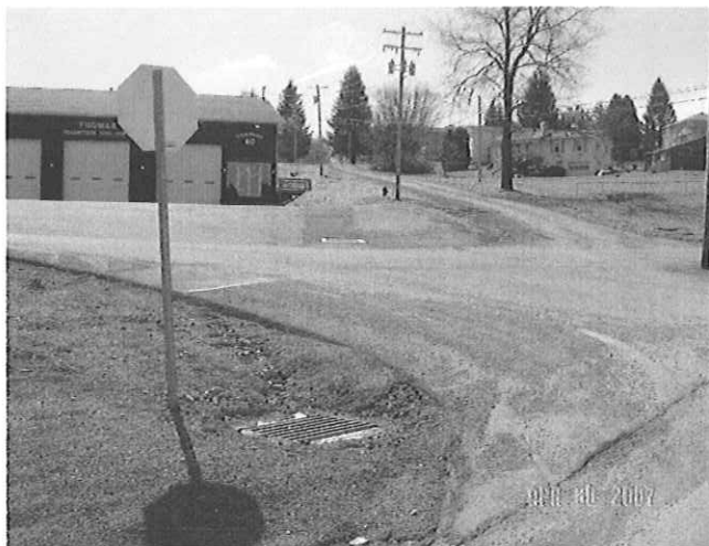
New Storm Drains and Catch Basins
