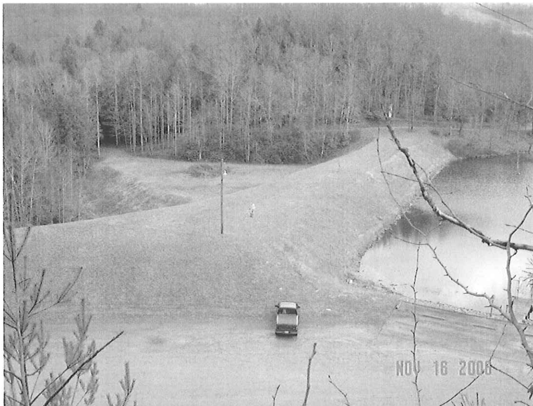
PLUM ORCHARD DAM MODIFICATION, FAYETTE CO., WV
