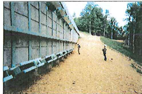
Finished wall with anchors
