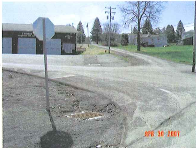
New Storm Drains and Catch Basins
