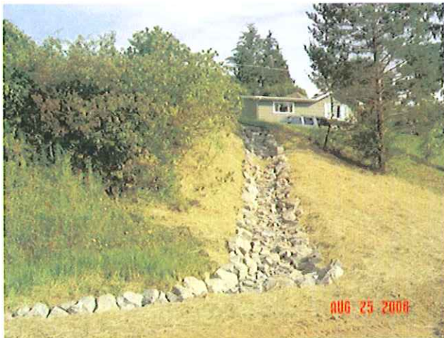
Erosion Repair – Rip Rap Armored Ditch
