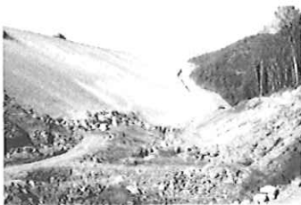
Cut and Fill King Coal Highway McDowell County
