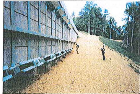
Finished wall with anchors
