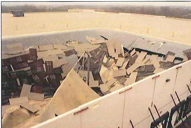
Roof Collapse
