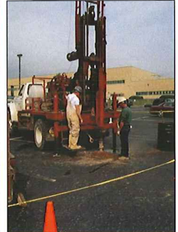
Drilling on Flat Terrain
