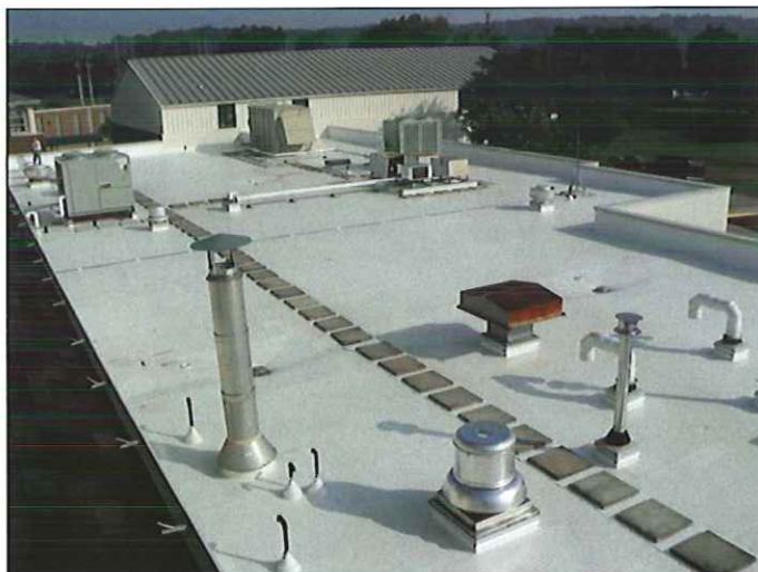
After Removal and Replacement
