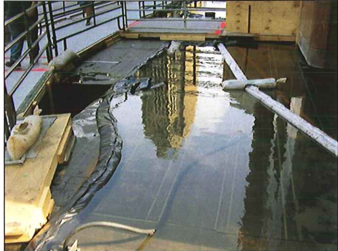
View of water flood test in progress to test for leakage
