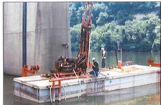
Barge Drilling
