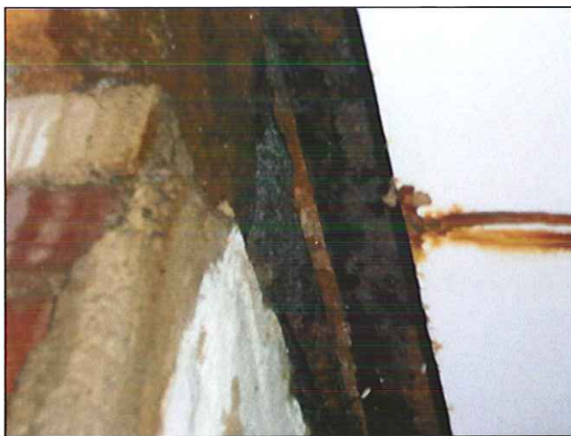
Corrosion due to moisture infiltration causing structural concern below the entryway
