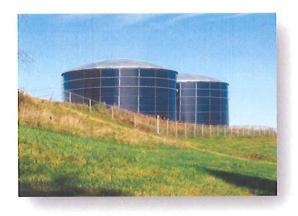
Contract 2 of this project included the construction of two (2) 522,000 gallon water storage tanks, including valve vault and piping, site work, access road, and fencing, complete, for the storage tanks.
