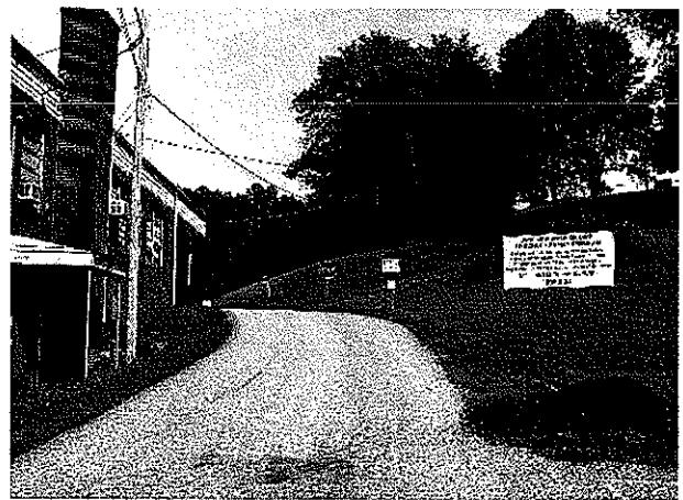
The terrain at Jane Lew Elementary School will require an elevated walkway to maintain separation from vehicles.
