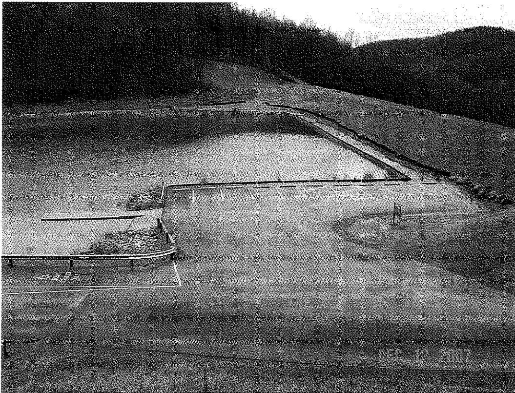
BAILEY DAM MODIFICATION, MONONGALIA CO., WV
