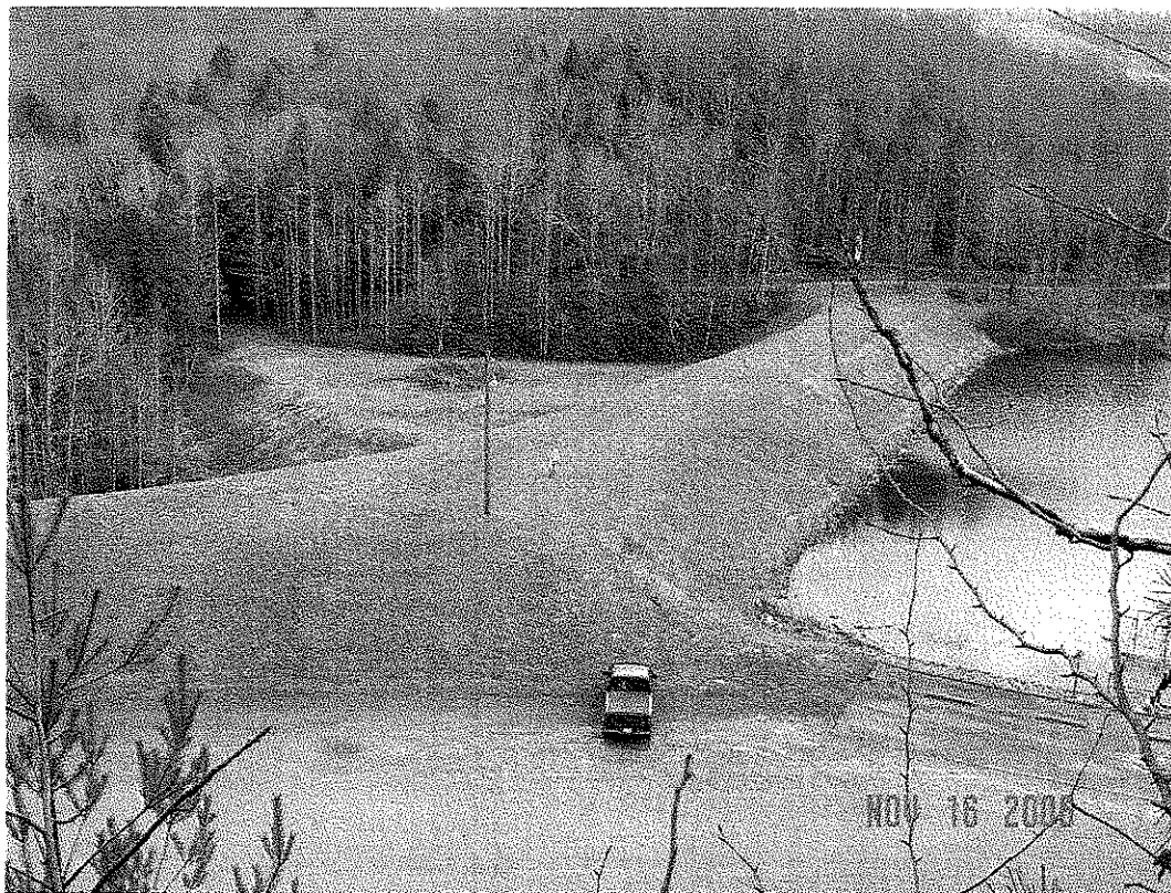
PLUM ORCHARD DAM MODIFICATION, FAYETTE CO., WV
