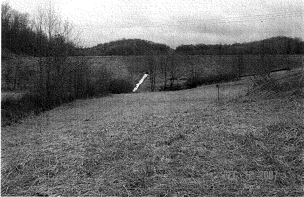
LEMLEY DAM MODIFICATION, MONONGALIA CO., WV
