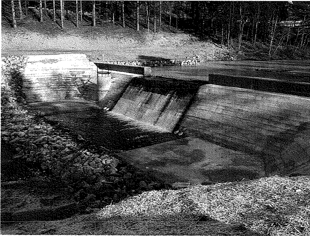
THOMAS DAM MODIFICATION, THOMAS, WV
