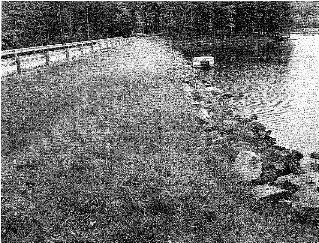
MONCOVE DAM MODIFICATION, MONROE CO., WV
