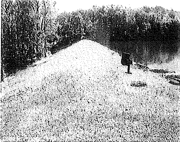
Photo No. 1: Dam crest facing right.
