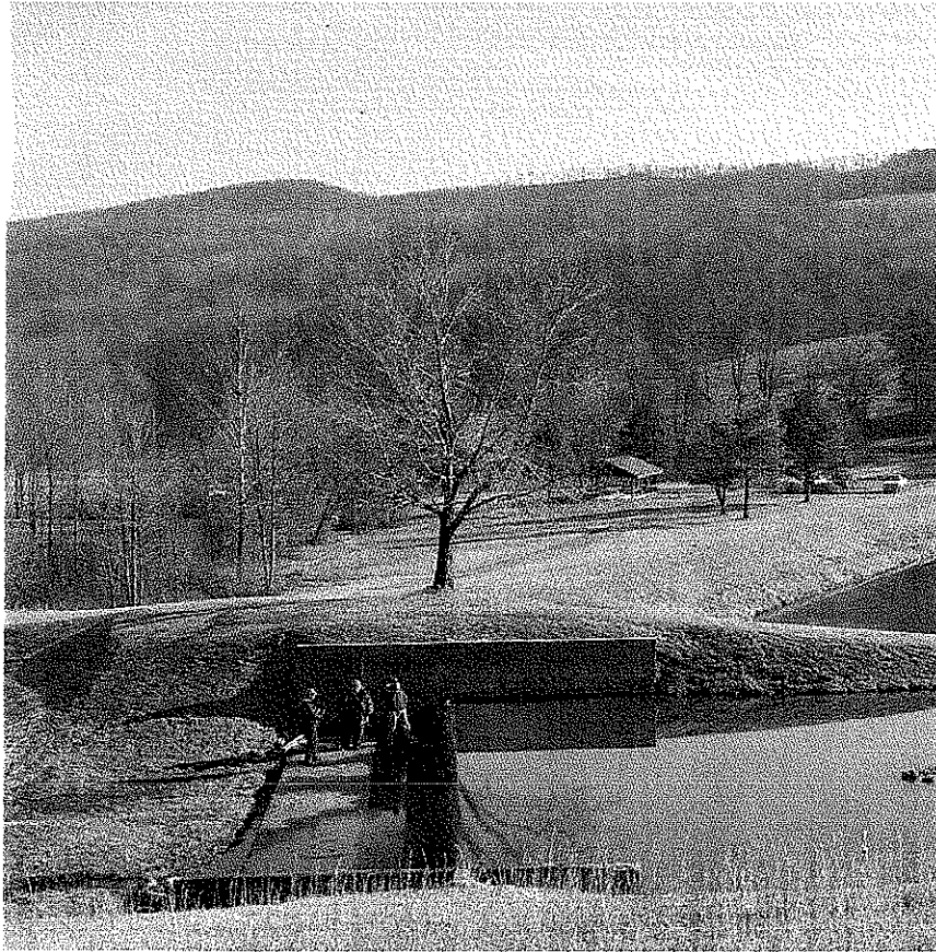
BELINGTON DAM MODIFICATION, BELINGTON, WV
