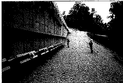
Finished wall with anchors
