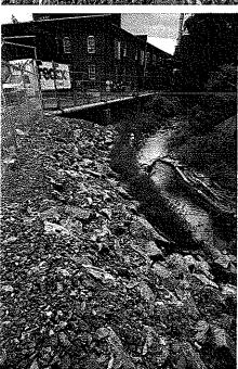
The overall proposed improvements consisted of re-alignment of the stream and the installation of rock vanes to redirect the flow so as to reduce near bank shear stress along the outside bend (previous location of gabion baskets). Other alternatives were investigated; however, concrete and gabion basket walls have been used in the past with a poor success rating.
