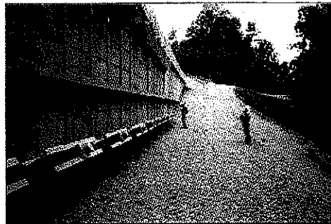
Finished wall with anchors
