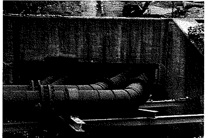
16-inch-diameter drainage pipes designed to convey water from mine shaft to existing treatment ponds.
