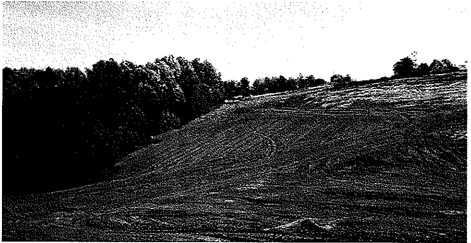
Black Dog Hollow site slope following regrading and removal of erosion features.
