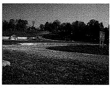
The project consisted of approximately 700 tons of asphalt base course, 350 tons of asphalt wearing course. crushed aggregate base course, drop inlet risers and existing concrete sidewalk removal and installation of handicap ramps. G&O is
