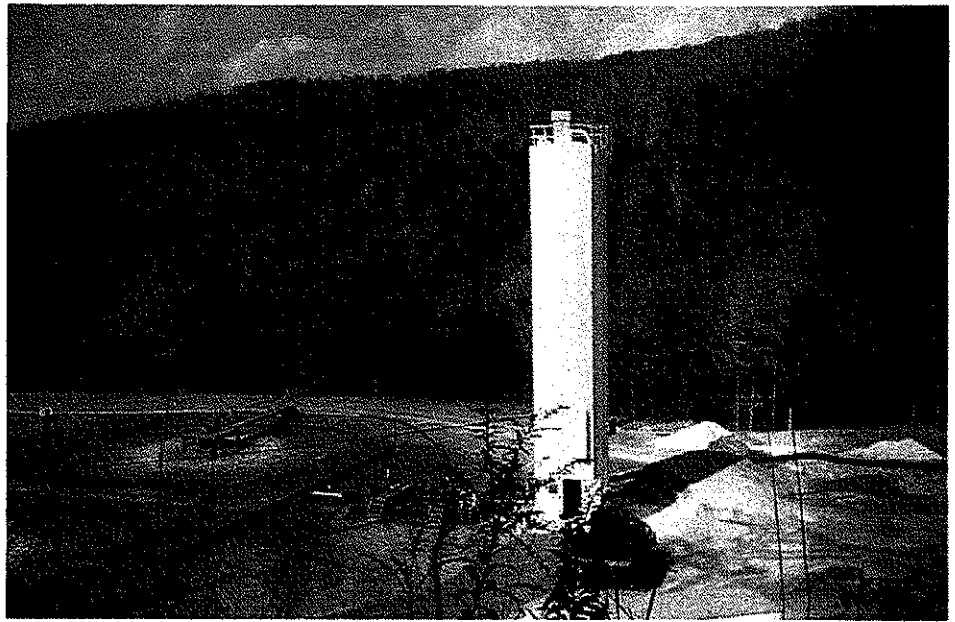
Lime storage bin, lime slaker and control unit, flash mix tank, and aeration system for treatment of AMD.
