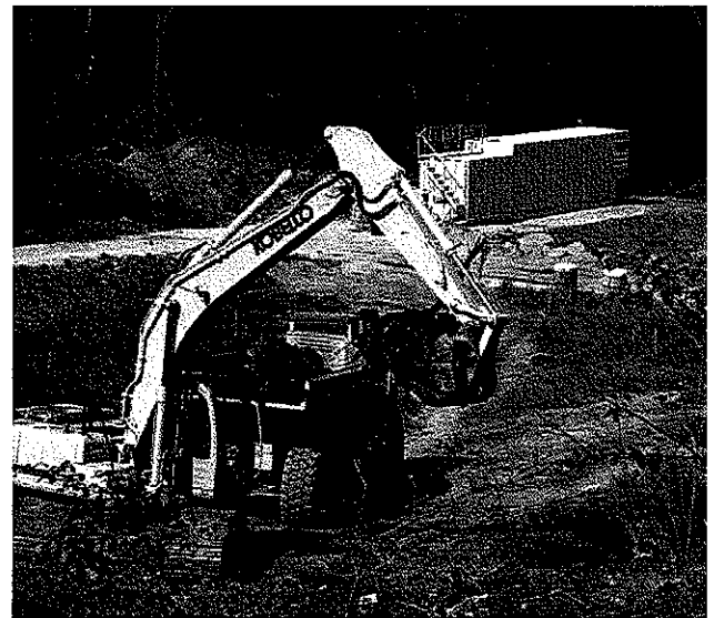
Removal of site waste for disposal at a nearby landfill.
