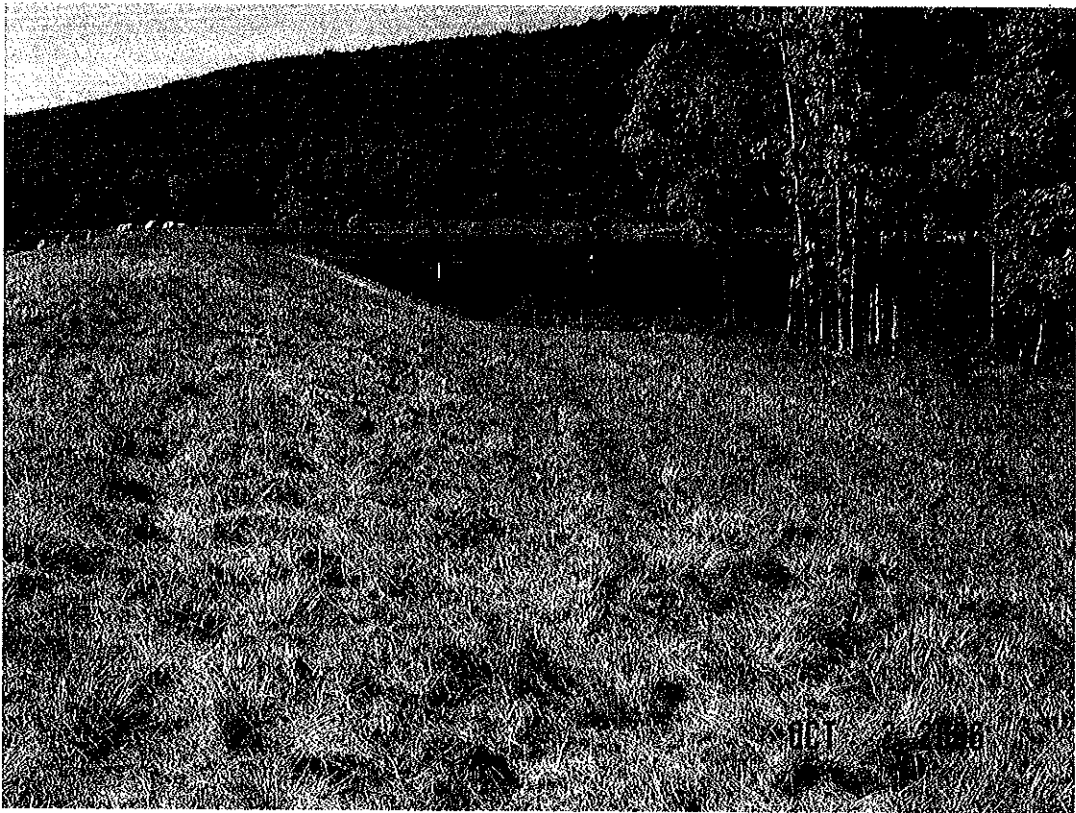
WARDEN LAKE DAM MODIFICATION, HARDY CO., WV
