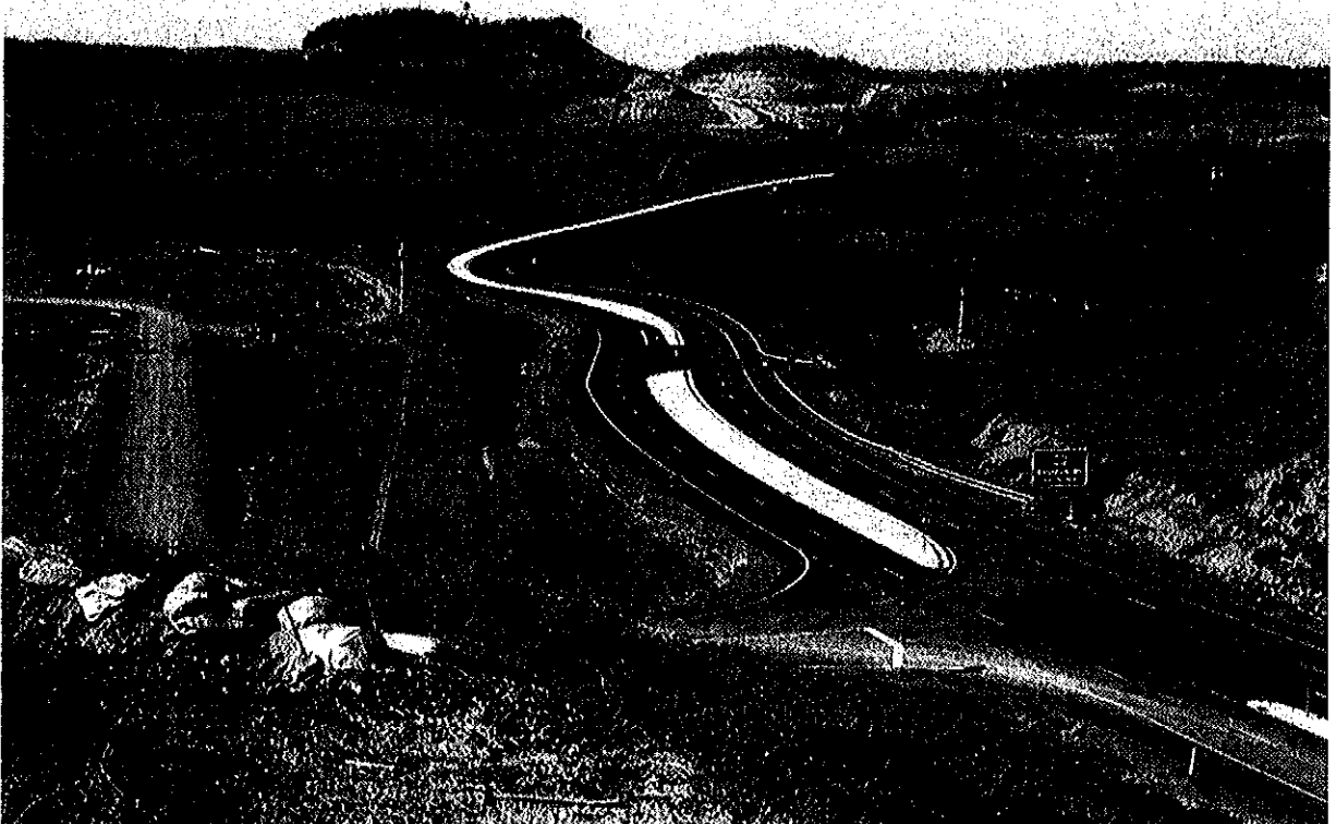
ROUTE 279, NORTH BRIDGEPORT BYPASS - COMPLETED IN 2000
