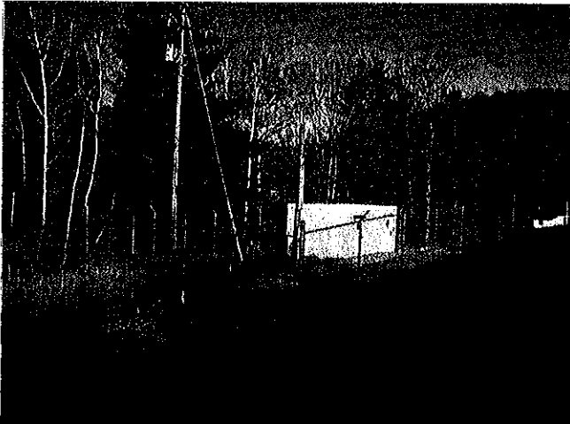
50 GPM Wilsontown Booster Station
