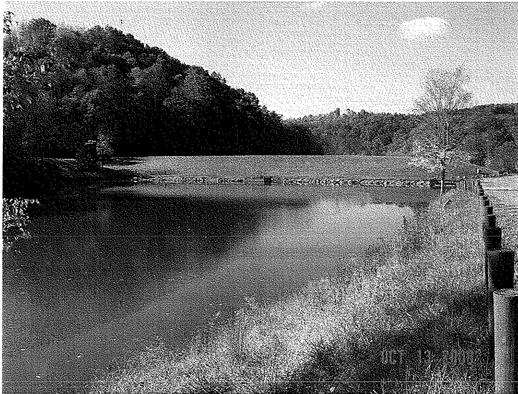
JIMMY LEWIS DAM MODIFICATION, MERCER CO., WV
