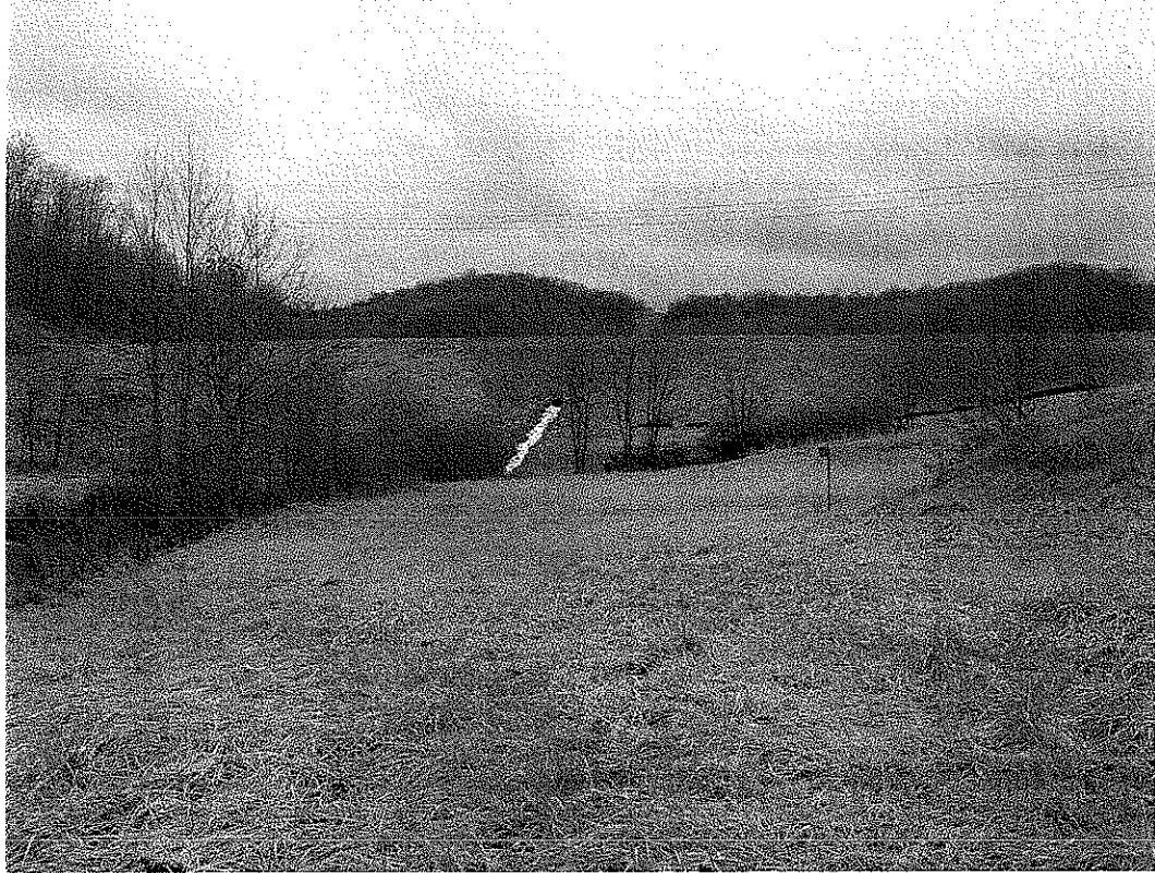
LEMLEY DAM MODIFICATION, MONONGALIA CO., WV
