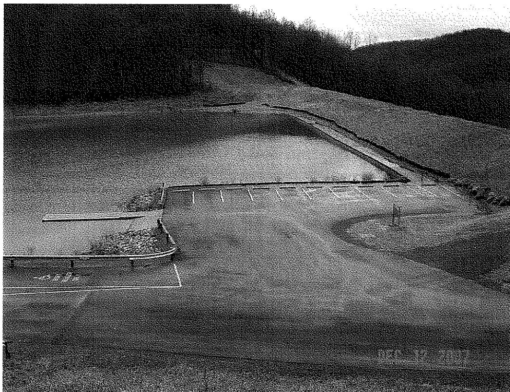
BAILEY DAM MODIFICATION, MONONGALIA CO., WV
