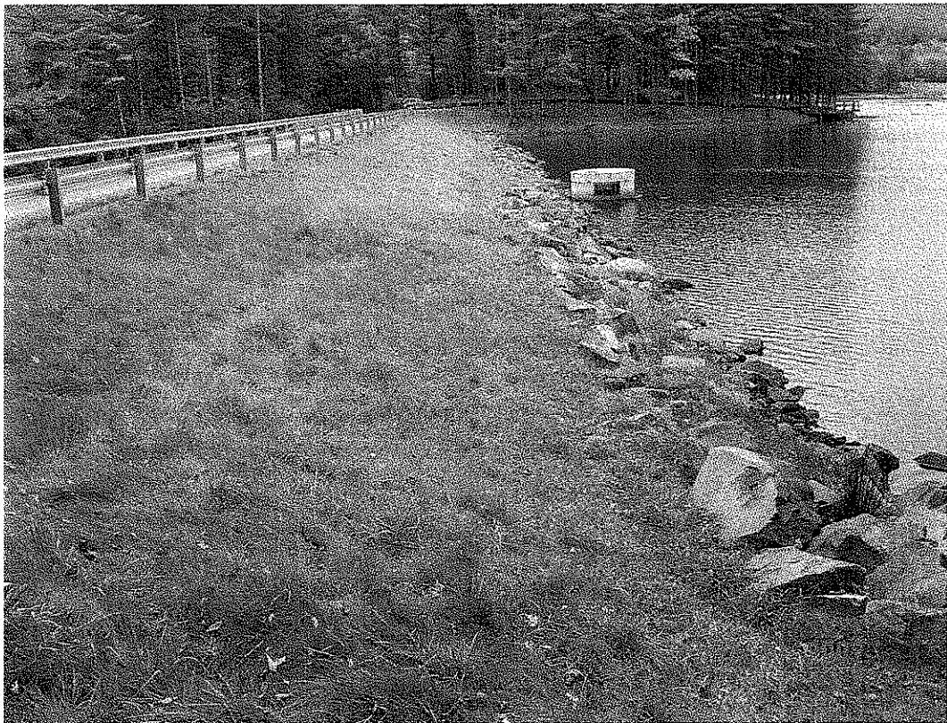
MONCOVE DAM MODIFICATION, MONROE CO., WV
