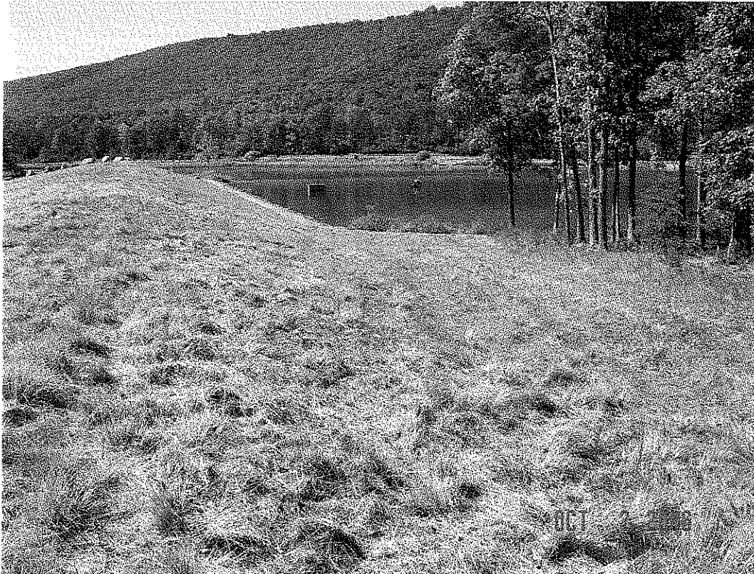
WARDEN LAKE DAM MODIFICATION, HARDY CO., WV
