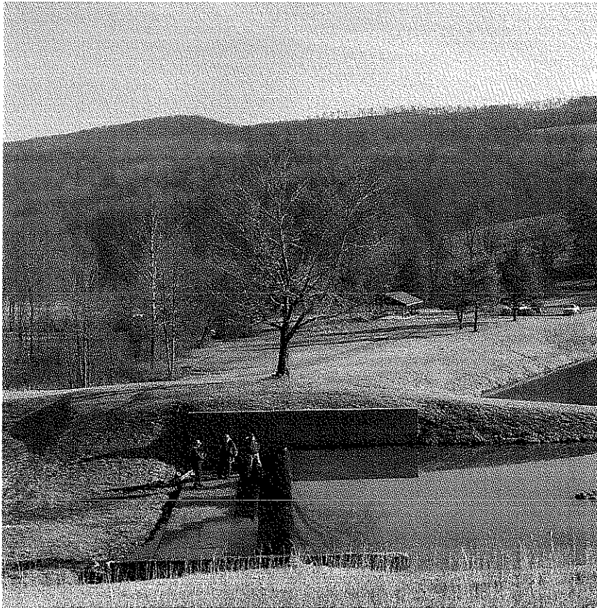
BELINGTON DAM MODIFICATION, BELINGTON, WV
