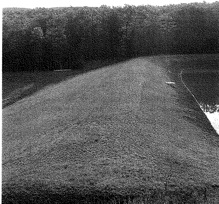
WILSON DAM MODIFICATION, HAMPSHIRE CO., WV
