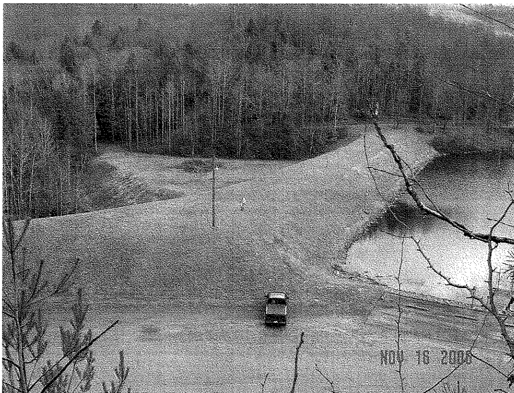
PLUM ORCHARD DAM MODIFICATION, FAYETTE CO., WV
