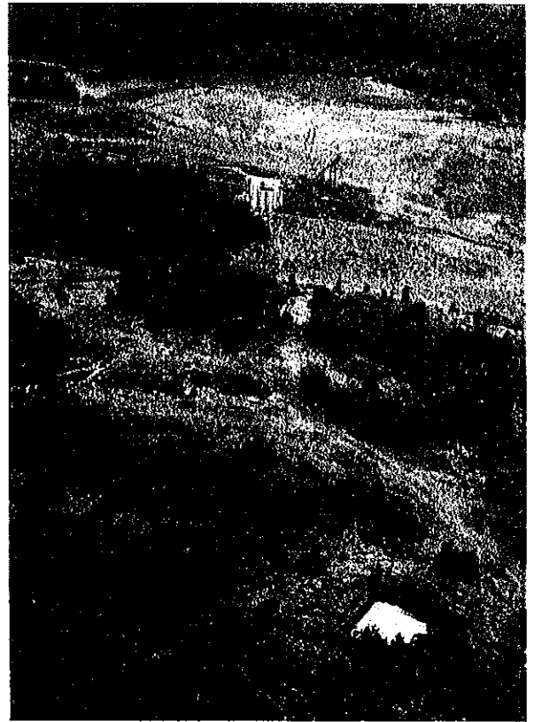
Aerial view of the Blackwood Mine Site at the time of the study. The building is an abandoned coal breaker. The square concrete pad in the foreground covers a deep ventilation shaft to the mine, but the sides of the pad partially collapsed, requiring further remediation.
