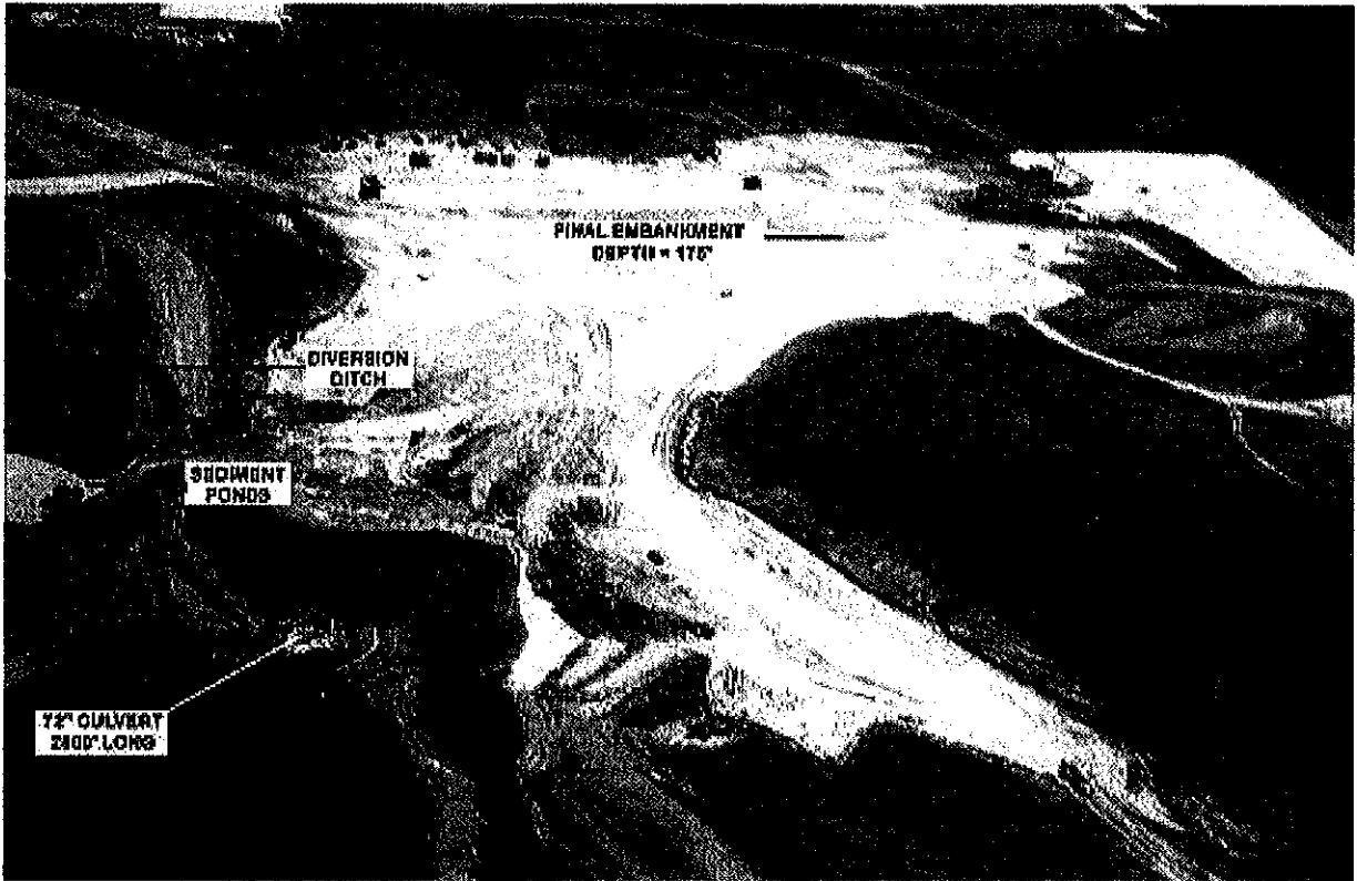
BENEDUM AIRPORT RUNWAY EXTENSION PROJECT - 1999
