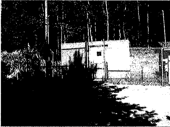
150 GPM Little Sand Run Booster Station
