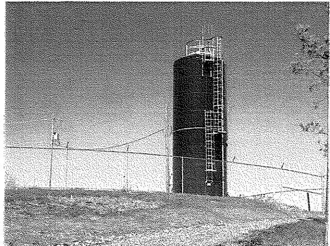
43,000 Gallon Salem Ridge Water Storage Tank
