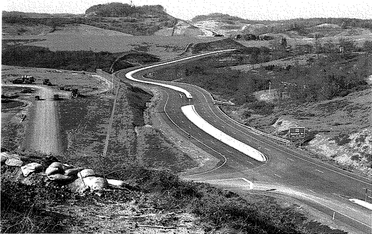
ROUTE 279, NORTH BRIDGEPORT BYPASS – COMPLETED IN 2000
