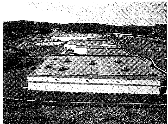
CTL Engineering of West Virginia, Inc. provided geotechnical engineering, materials testing, observation services and surveying services for this project.
