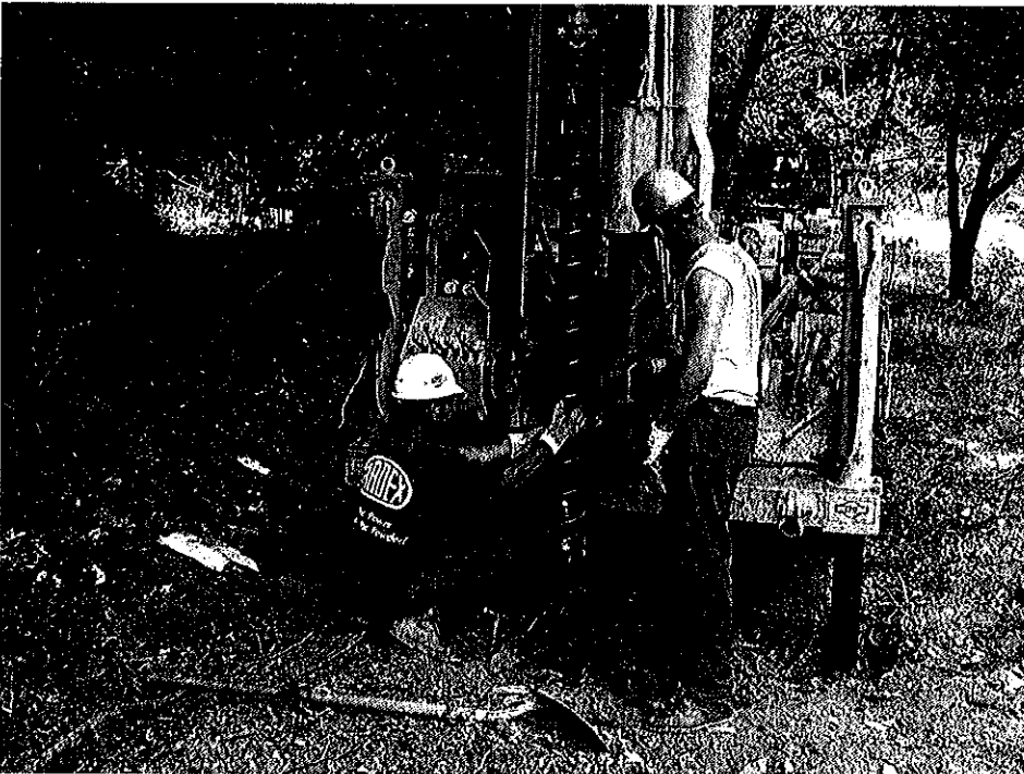
Drilling and sampling performed as part of the D'Appolonia field exploration program.
