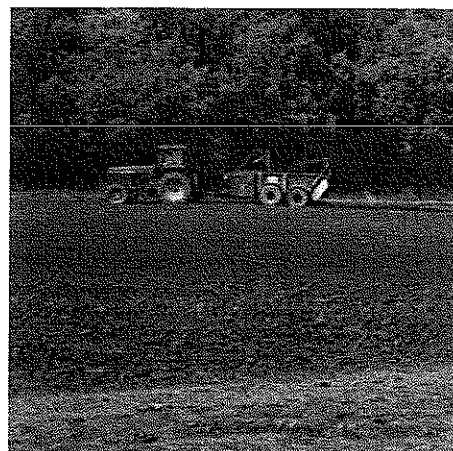
Application of biosolids to regraded site.
