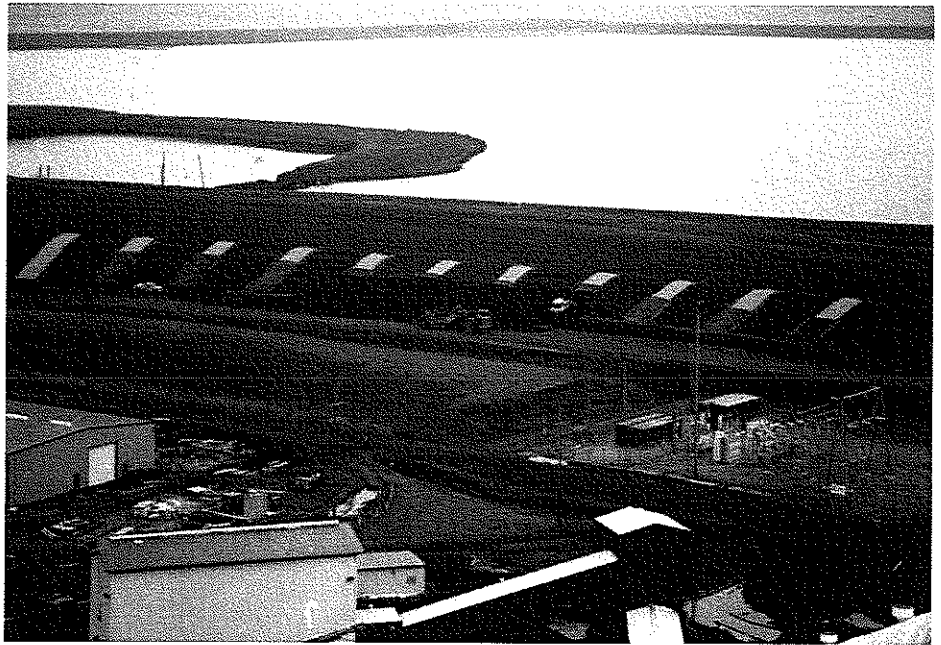
Finger drains under construction at coal refuse disposal facility in Illinois.
