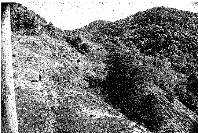
ORIGINAL NORTH REFUSE AREA
